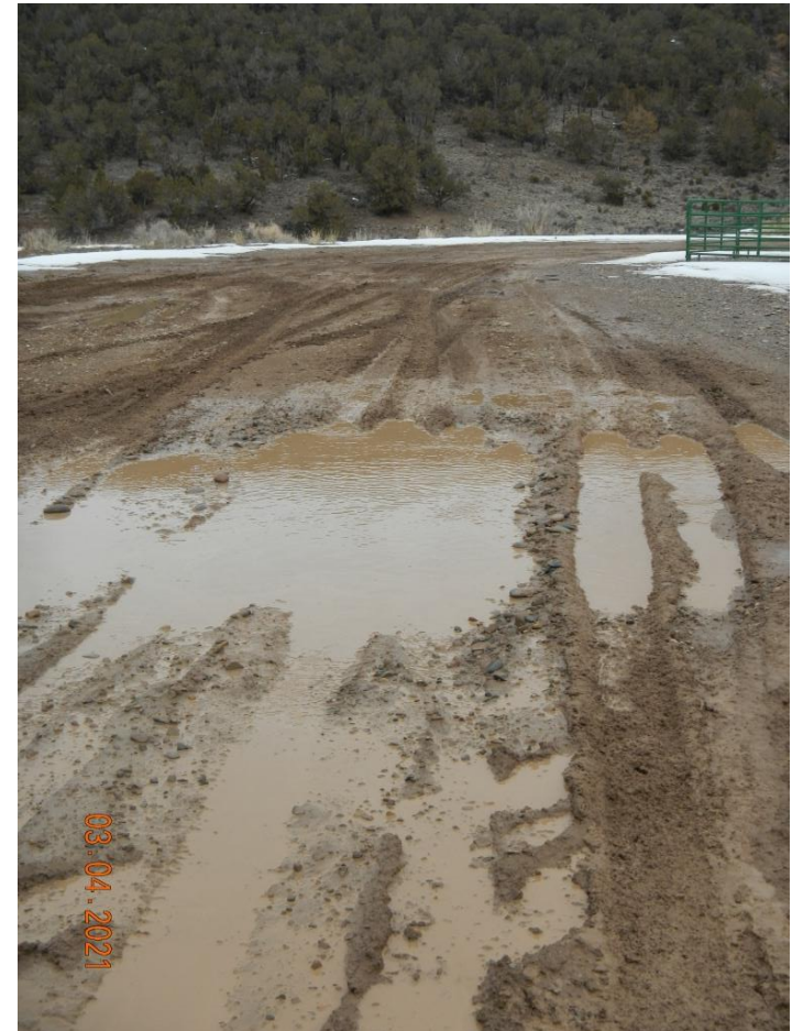
Photo#4: Rutting/ponding on Pad.
