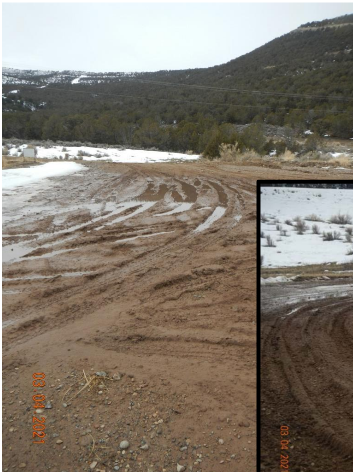
Photo#3: Rutting at entry and in traffic patterns.
