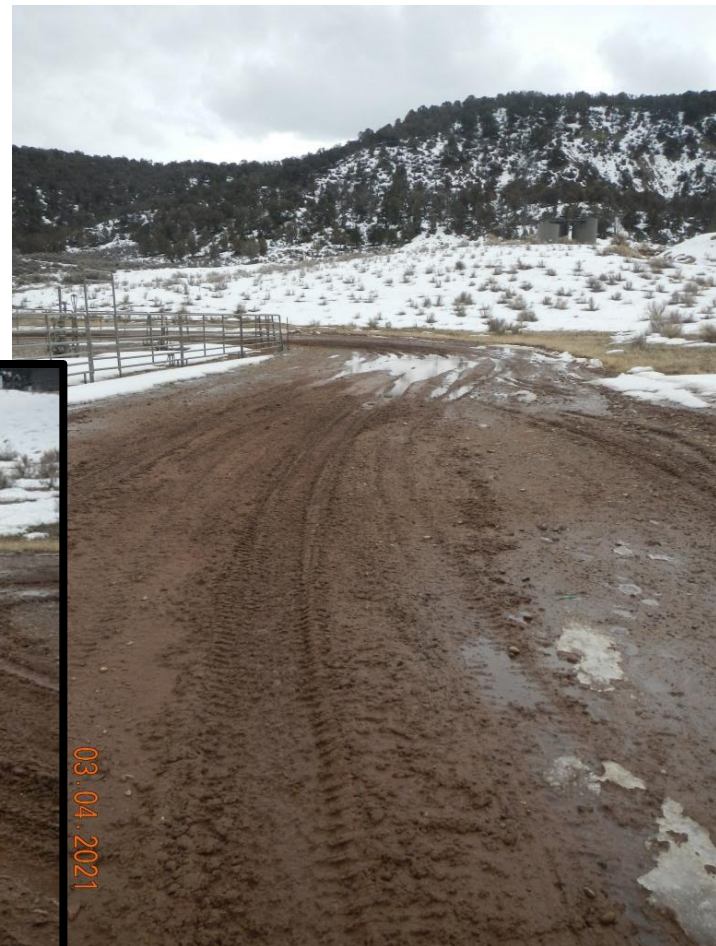
Photo#4: Rutting at entry and in traffic patterns.
