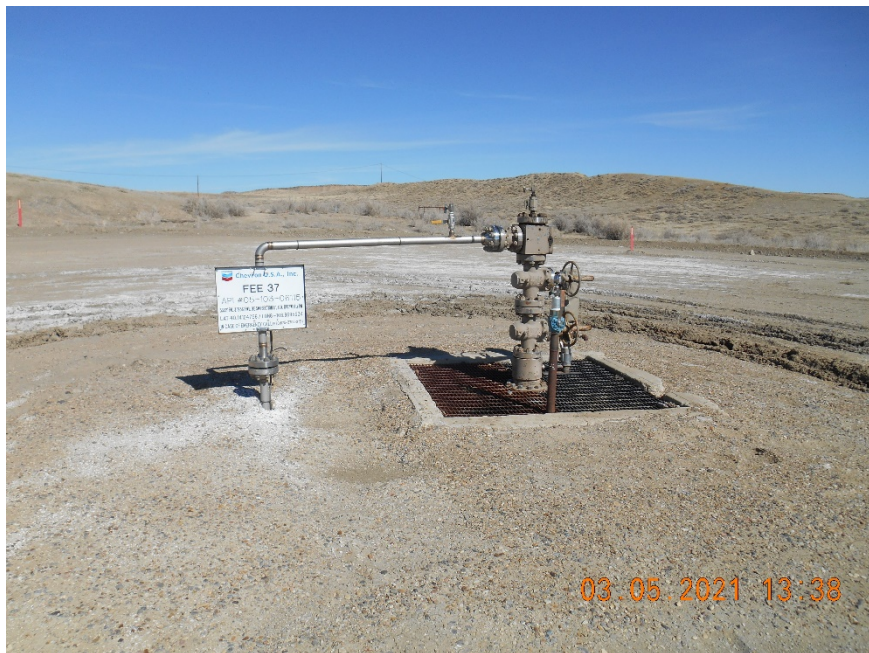
Injection wellhead
