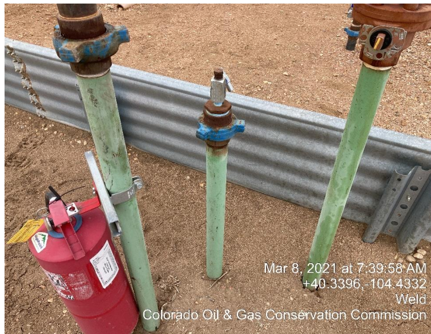
Photo #23 Unmarked or LO/TO Riser
