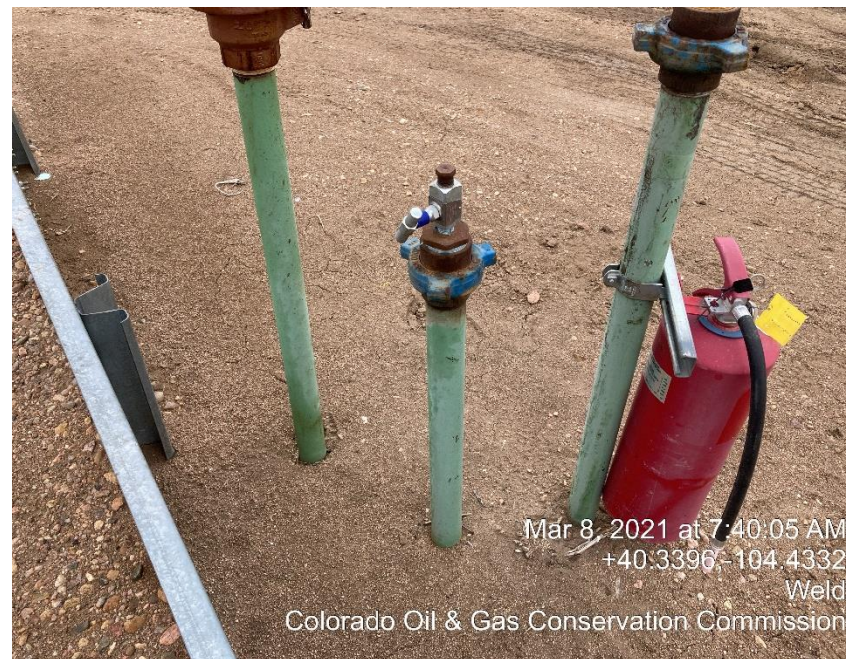
Photo #24 Unmarked or LO/TO Riser
