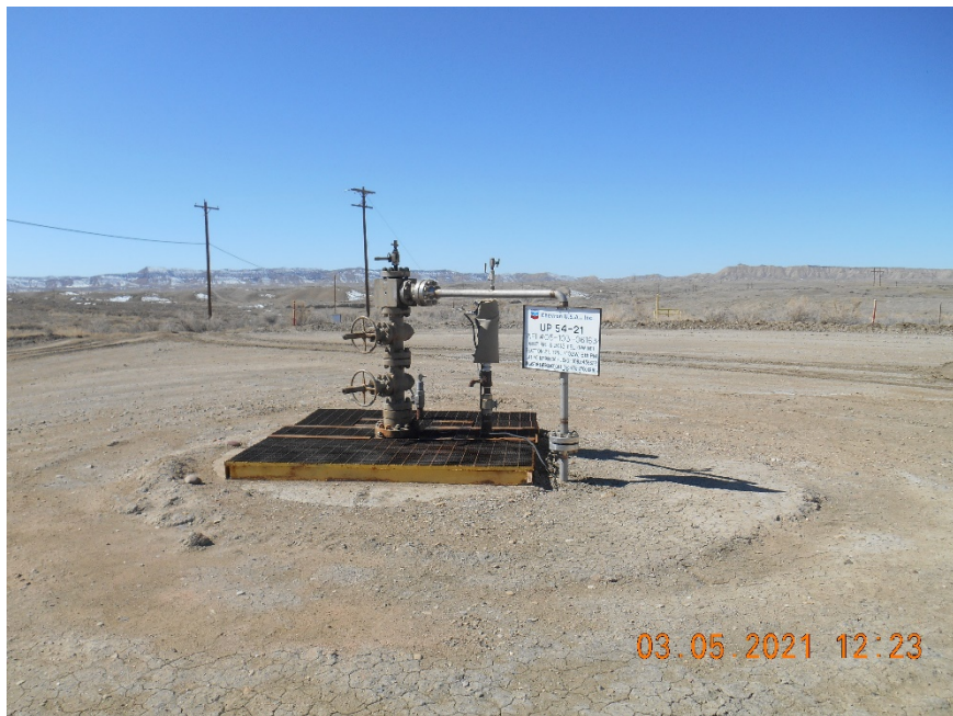
Injection wellhead
