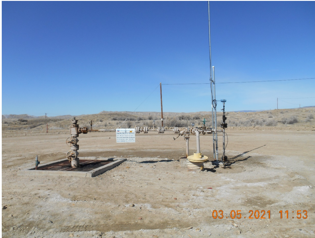
Injection wellhead
