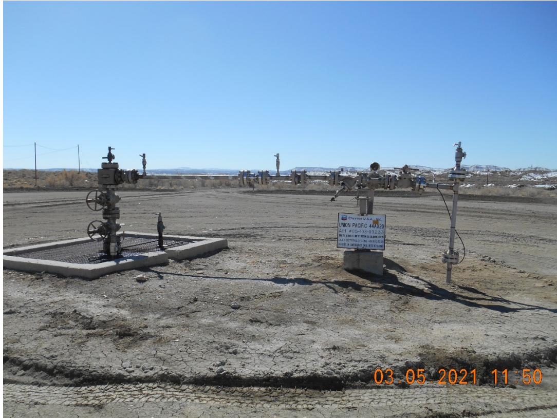
Injection wellhead
