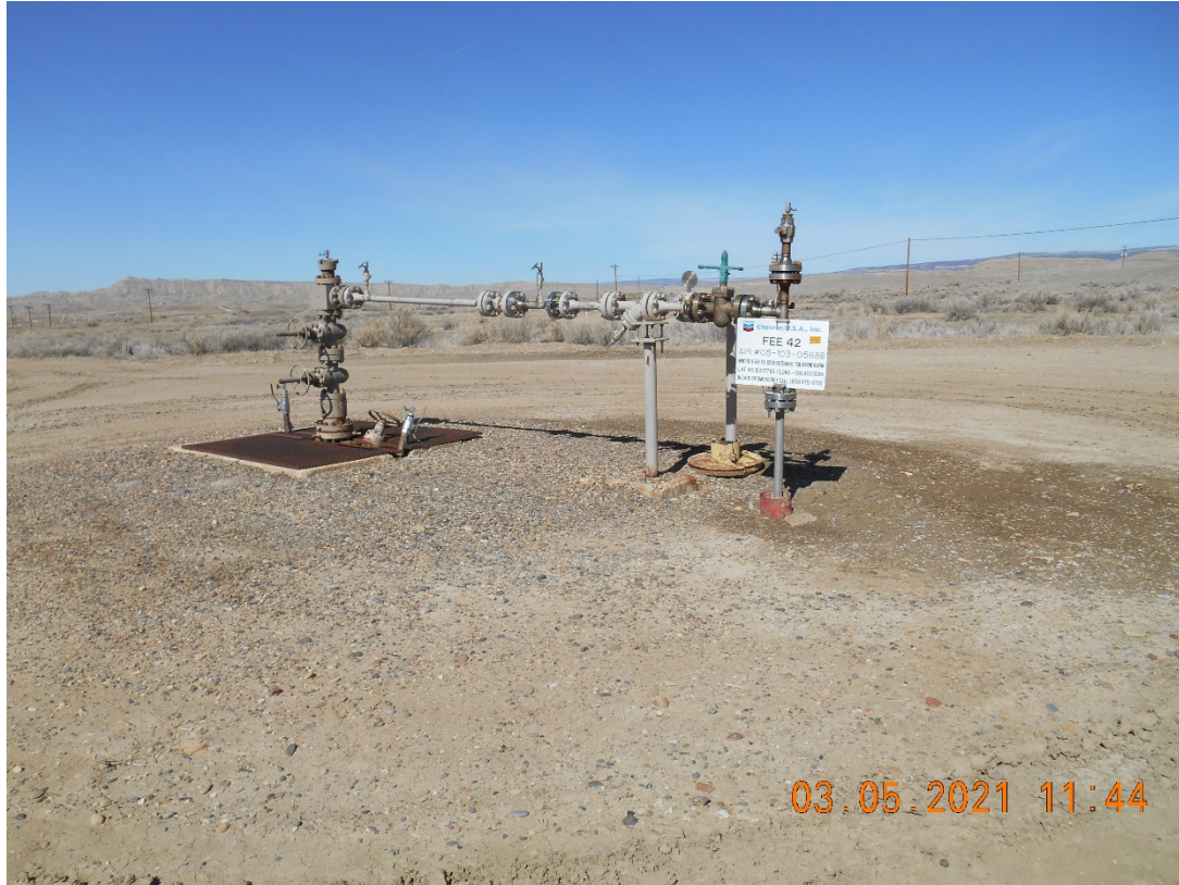
Injection wellhead- Temporarily Abandoned
