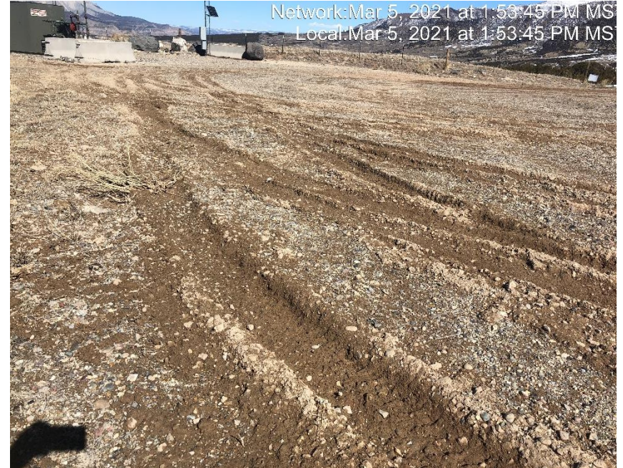
Photo #3073 Rutting present on location due to lack of stabilization.
