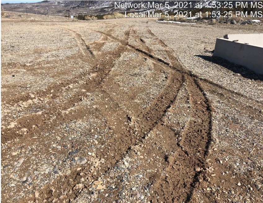
Photo #3072 Rutting present on location due to lack of stabilization.
