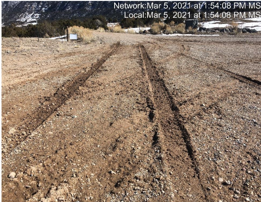
Photo #3074 No form of tracking control.
