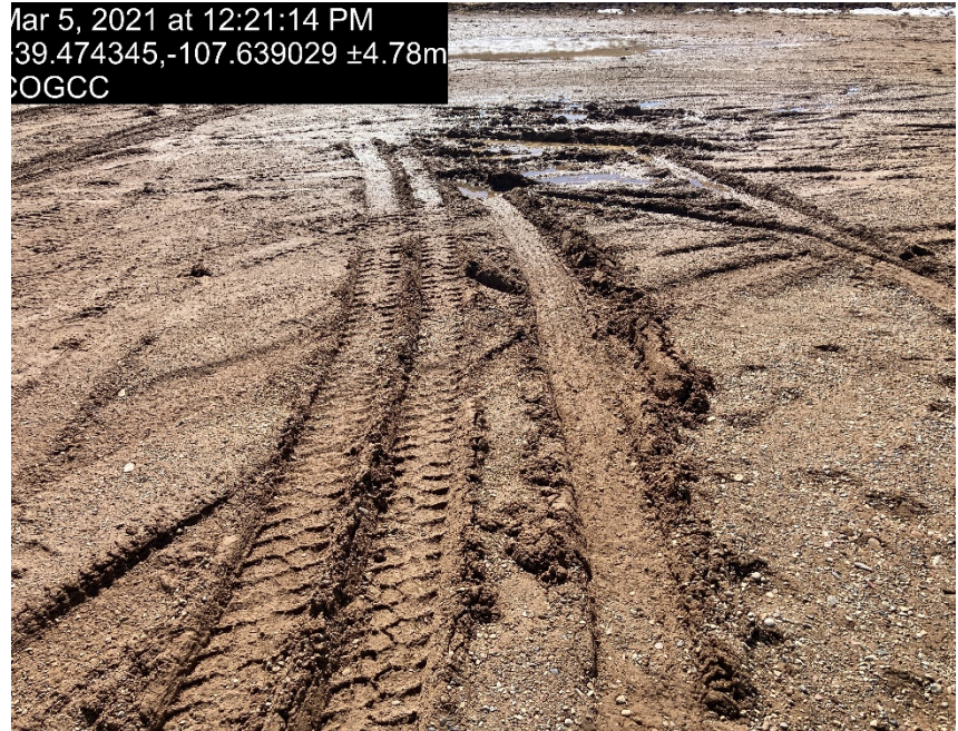
Lack of stabilization/compaction
