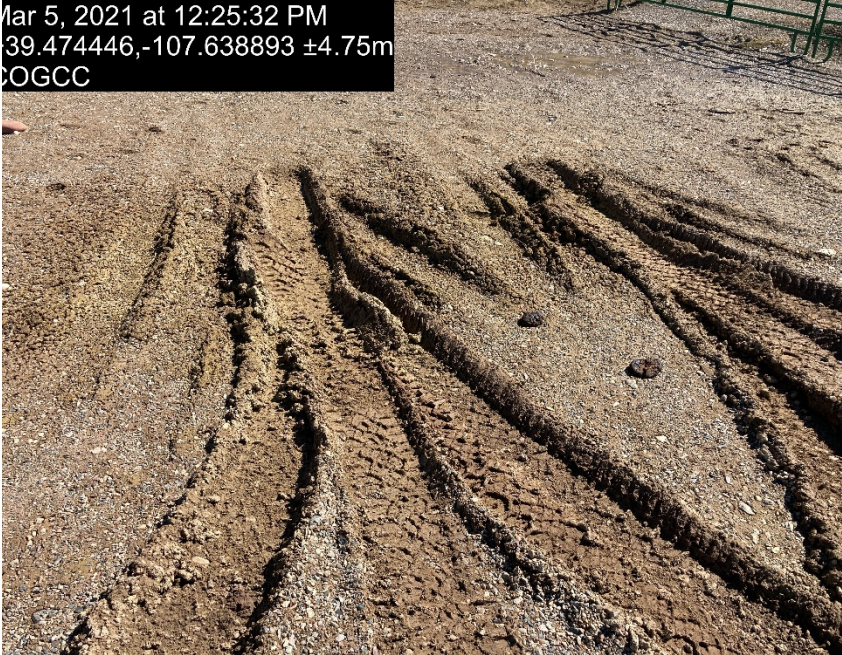
Lack of stabilization/compaction
