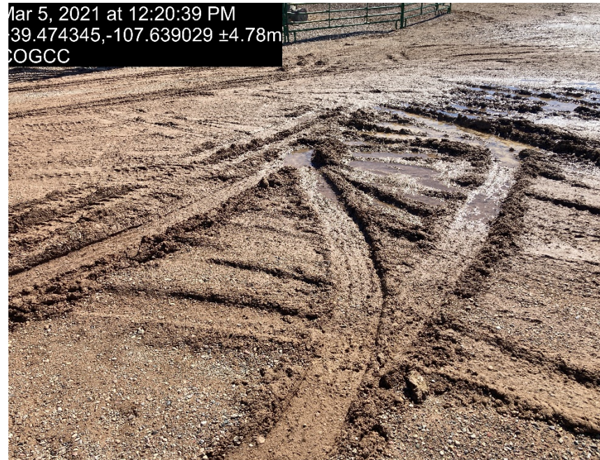
Lack of stabilization/compaction
