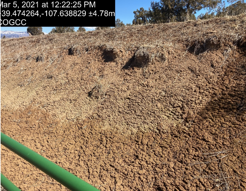
Cut slope on East side of location shows evidence of erosion/not stabilized
