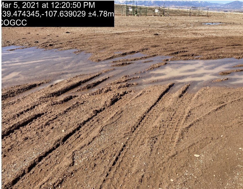
Lack of stabilization/compaction
