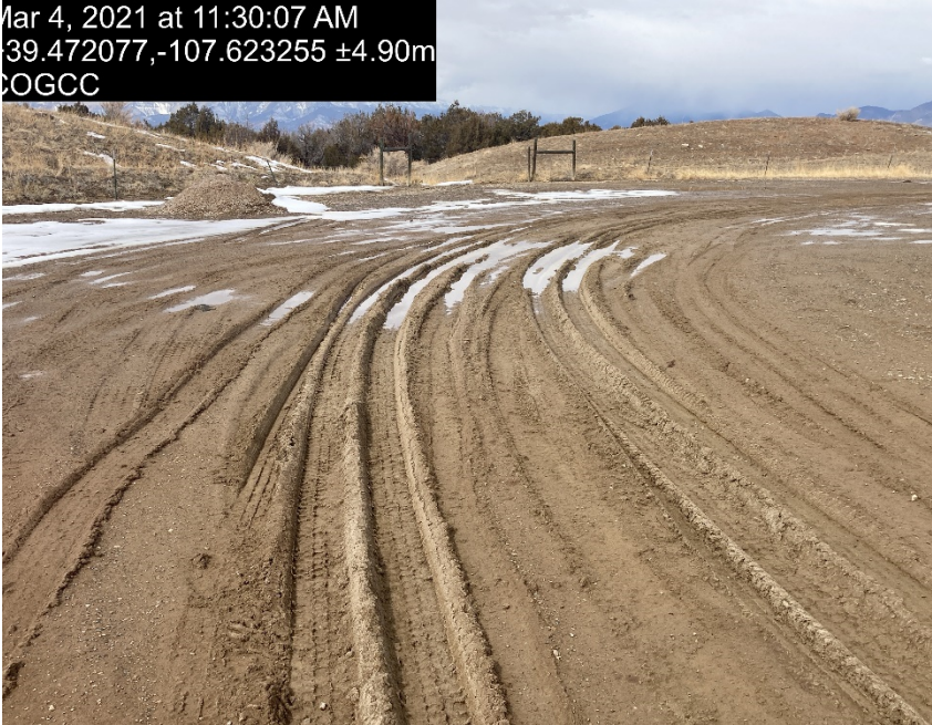
lack of stabilization/compaction
