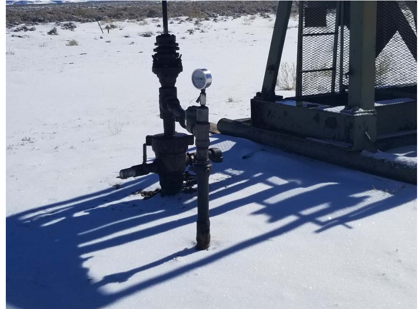
Photo 2. No bradenhead access apparent.
