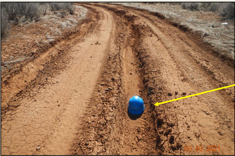
Photos 3/4. View of rutting and tracking up to 15 inches deep and wide observed along the access road.
