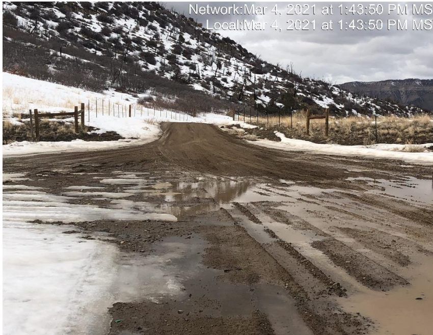
Photo #3049 No form of tracking control at entrance to location.
