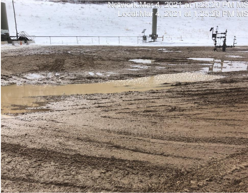
Photo #3047 Rutting present on location due to lack of stabilization.
