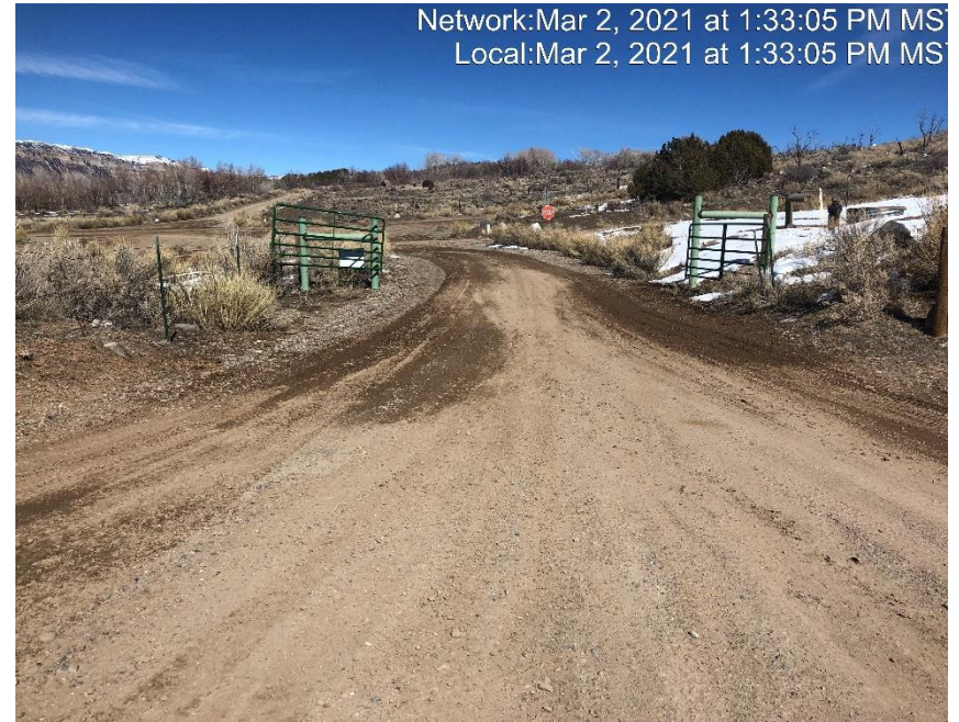
Photo #3040 No form of tracking control at entrance to location
