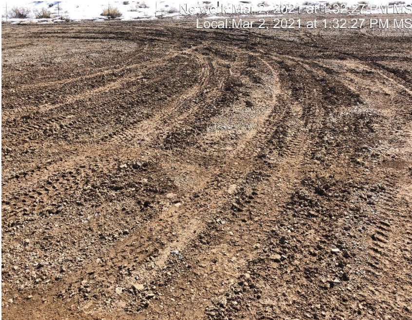
Photo #3038 Rutting present on location due to lack of stabilization
