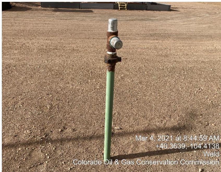
Photo #3 Unmarked riser
