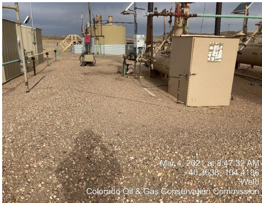
Photo #9 Weathered berm
