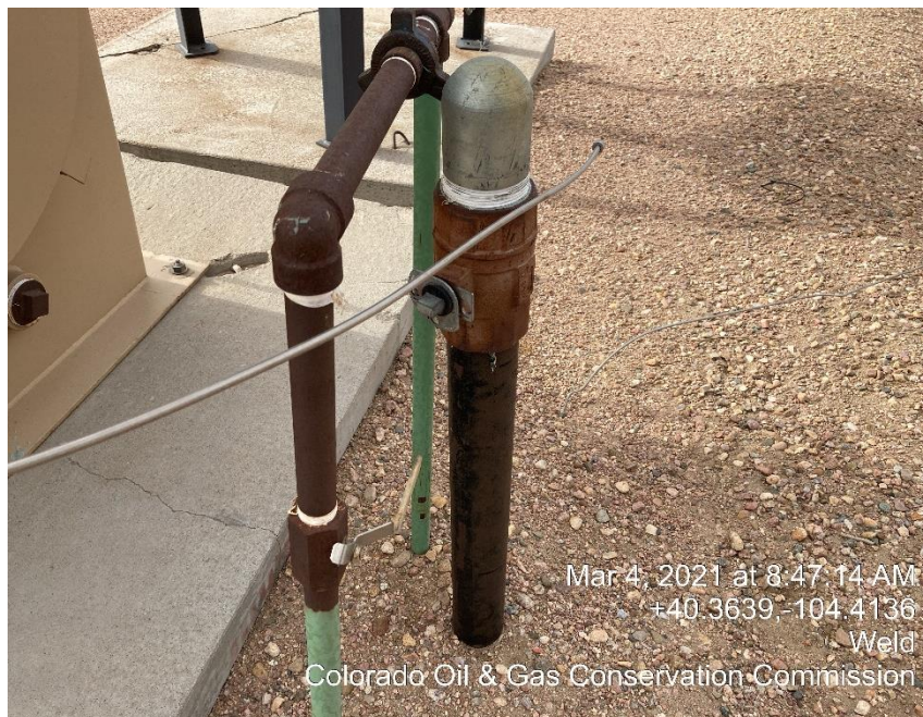
Photo #13 Unmarked riser and not LO/TO. Unused stainless line
