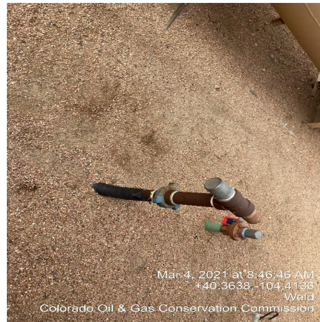
Photo #12 Unmarked riser
