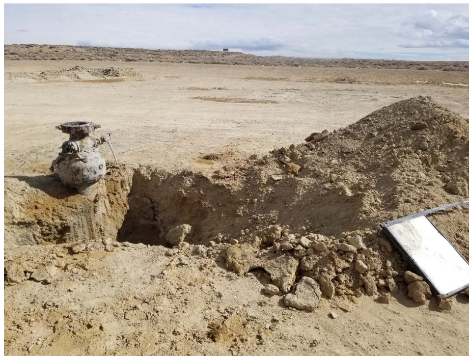
Photo 1. Well waiting for cut and cap.
