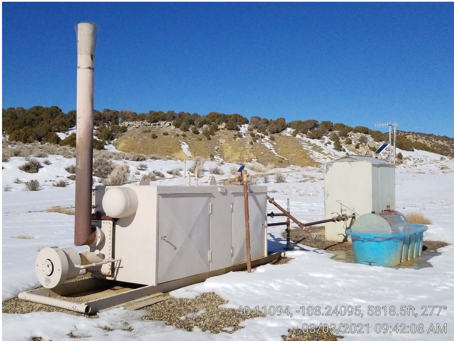
Photo 3. Separator & meter building.
