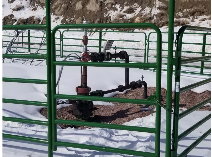
Photo 2. No bradenhead access apparent.
