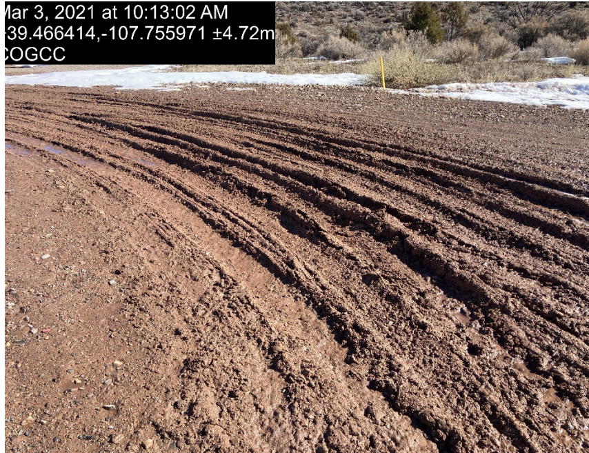
Lack of stabilization/compaction
