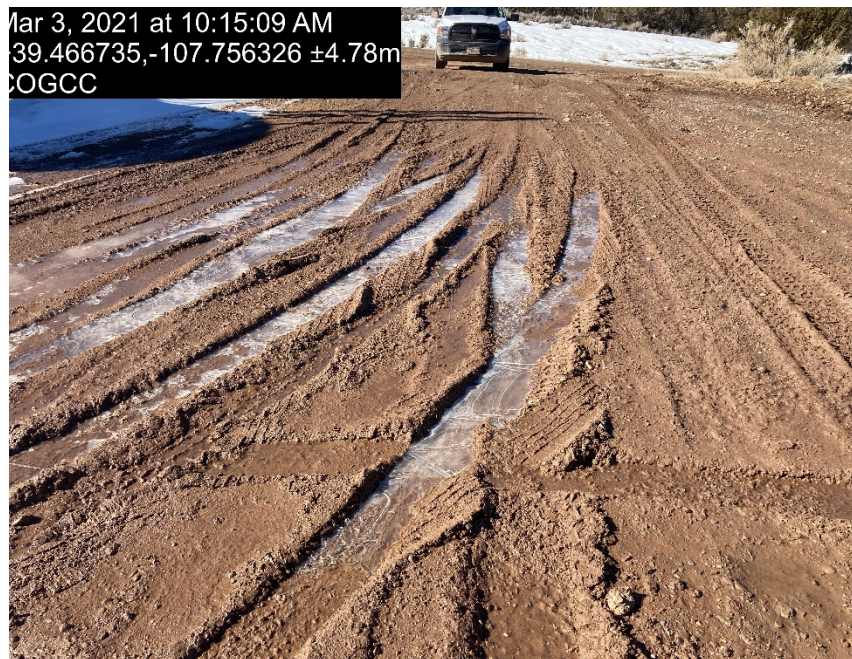
Lack of stabilization/compaction
