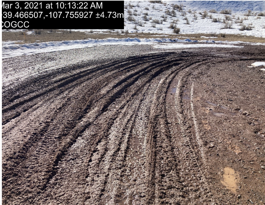
Lack of stabilization/compaction
