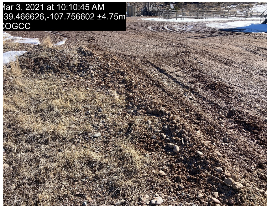
Sediment/berm plowed off of location
