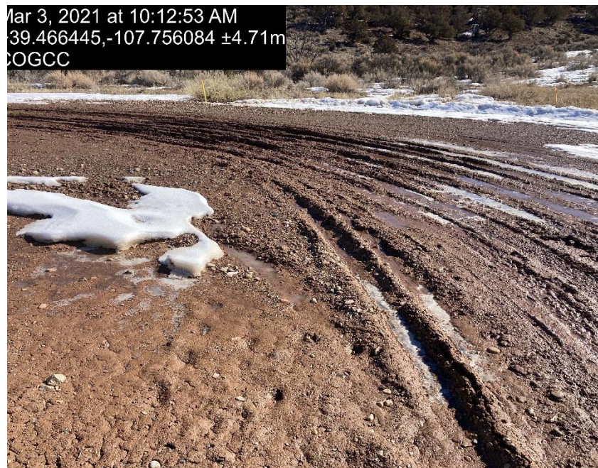
Lack of stabilization/compaction
