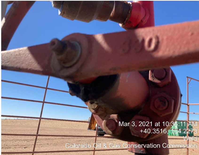
Photo #14 Leaking Master valve “mechanical conditions”
