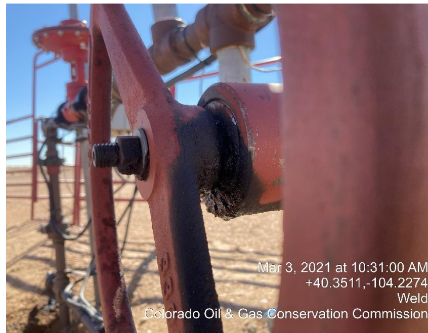
Photo #7 Leaking master valve "Mechanical Conditions"
