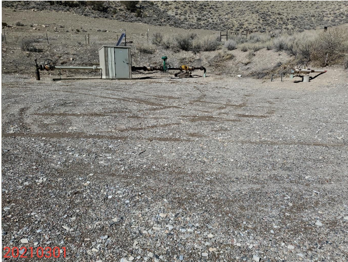
Photo 8: Photo taken from the southern areas of the Location, facing west. Photo shows lower section of the Pad. Production areas have been stabilize with gravel; not immediate stormwater concerns observed.
