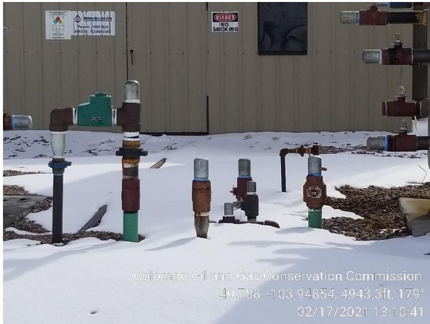
Photo 5 – Unmarked Risers
