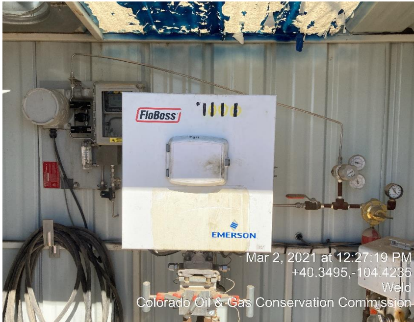
Photo #66 Missing Gas Meter Calibration Card
