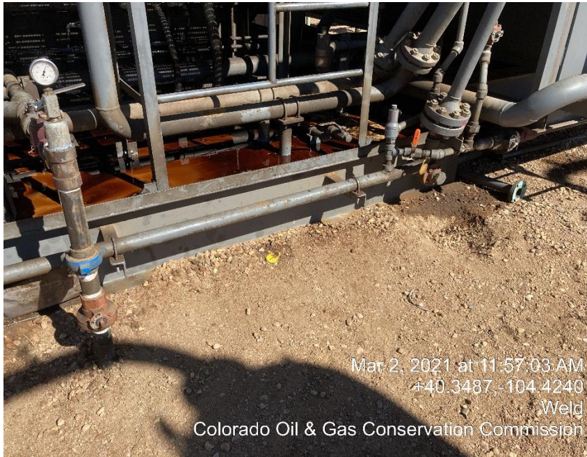
Photo #23 Stained soil/ Oily skid
