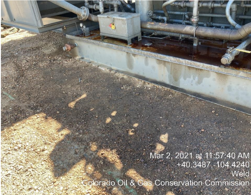
Photo #27 Stained soil/ Oily skid
