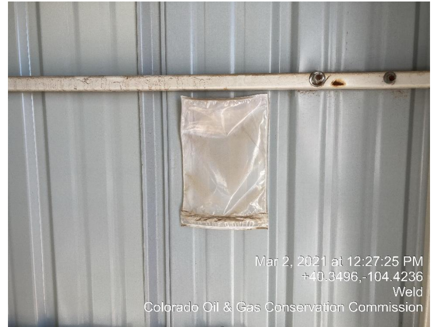
Photo #67 Missing Gas Meter Calibration Card
