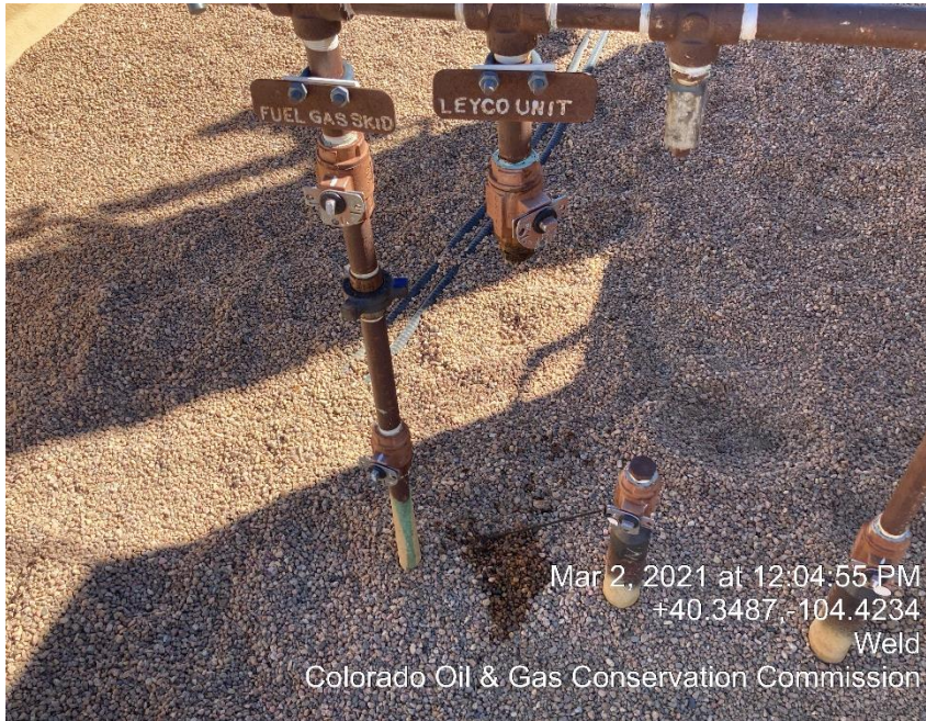
Photo #59 Mechanical Conditions/ Stained soil
