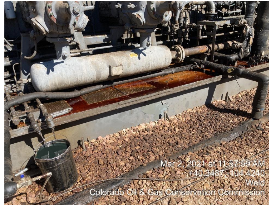
Photo #30 Stained soil/ Oily waste in bucket/ Oily skid
