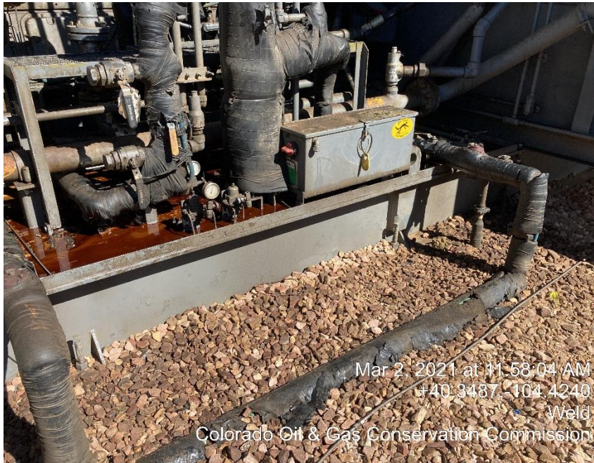
Photo #31 Stained soil/ Oily skid
