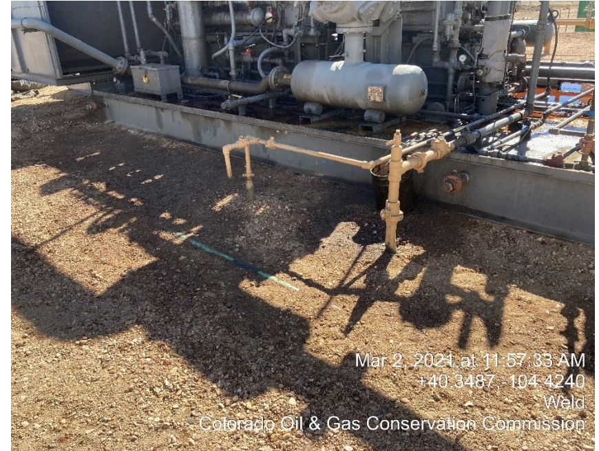
Photo #26 Stained soil/ Oily skid
