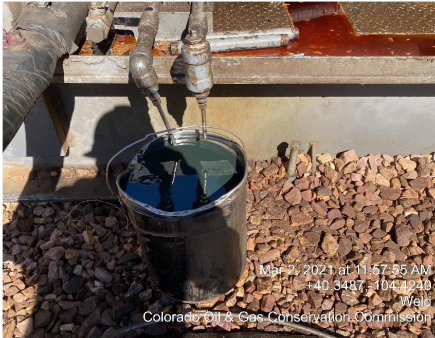
Photo #29 Stained soil/ Oily waste in bucket/ Oily skid
