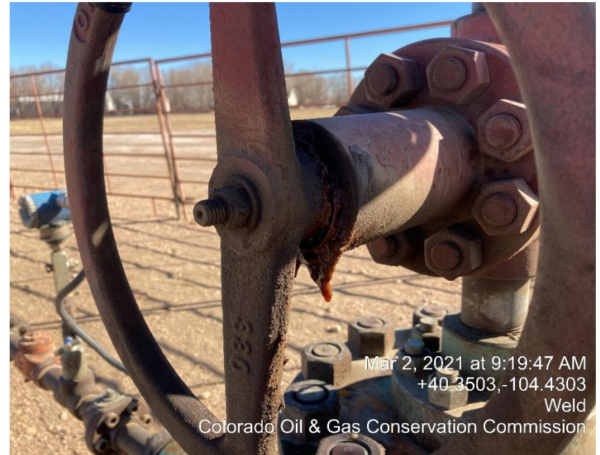
Photo #12 Leaking Master Valve
