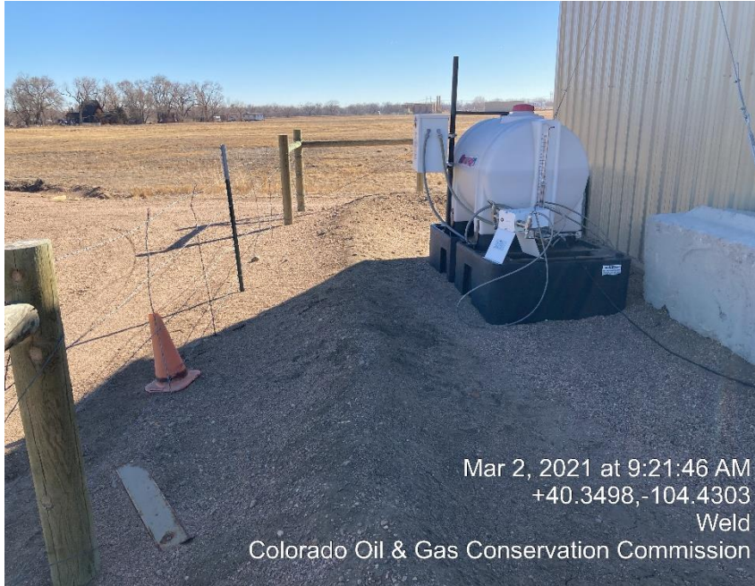
Photo #25 Weathered Berm
