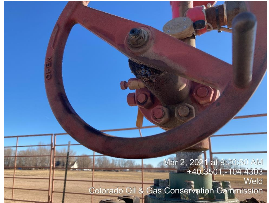
Photo #18 Leaking Master Valve
