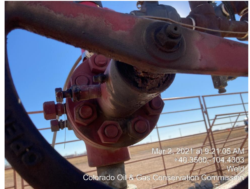
Photo #20 Leaking Master Valve
