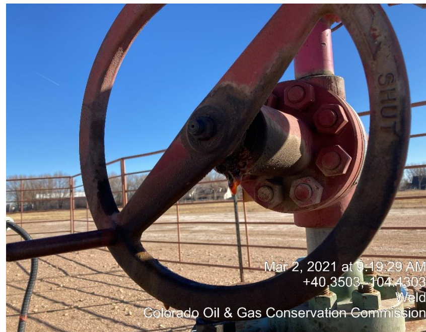
Photo #10 Leaking Master Valve
