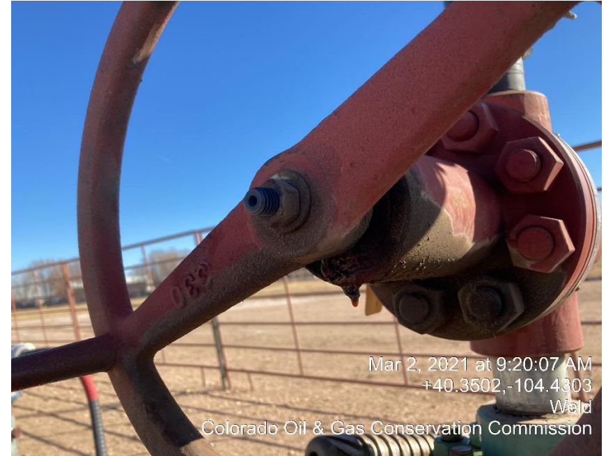
Photo #14 Leaking Master Valve
