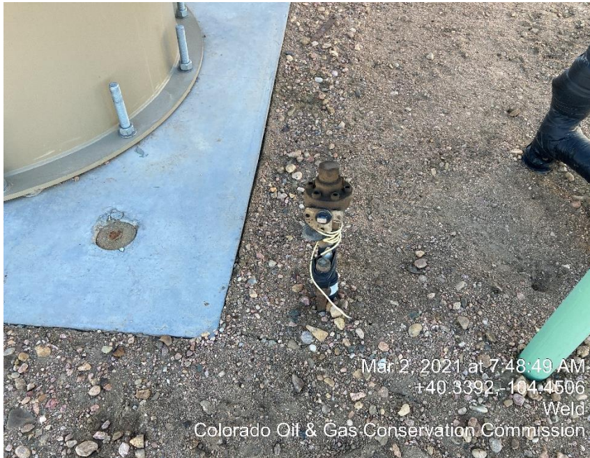
Photo #10 Unmarked Riser
