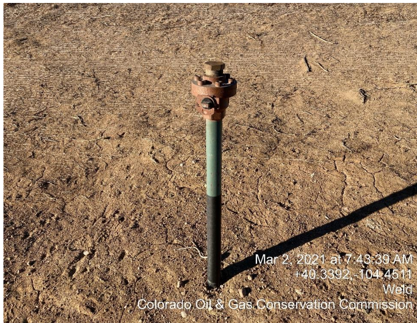
Photo #6 Unmarked Riser
