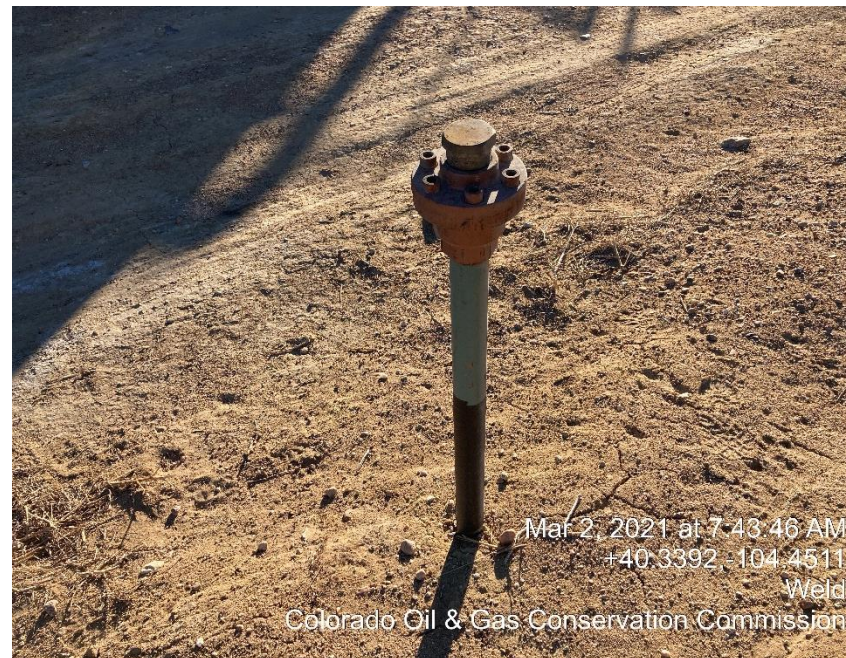
Photo #7 Unmarked Riser
