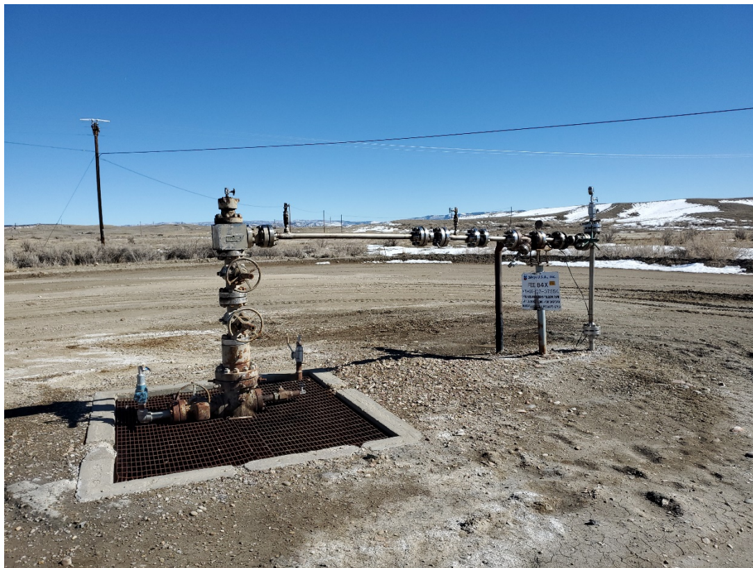
Injection wellhead
