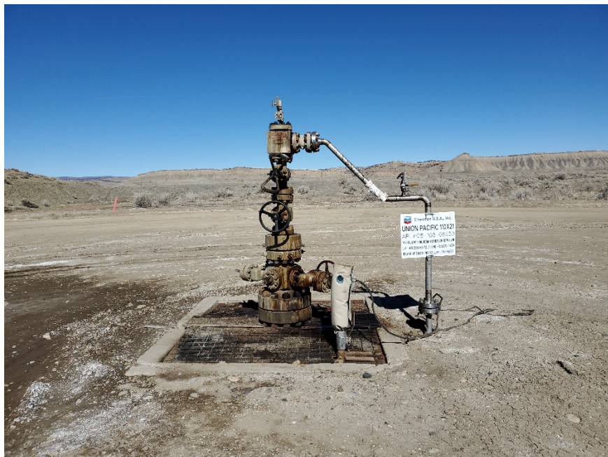
Injection wellhead
