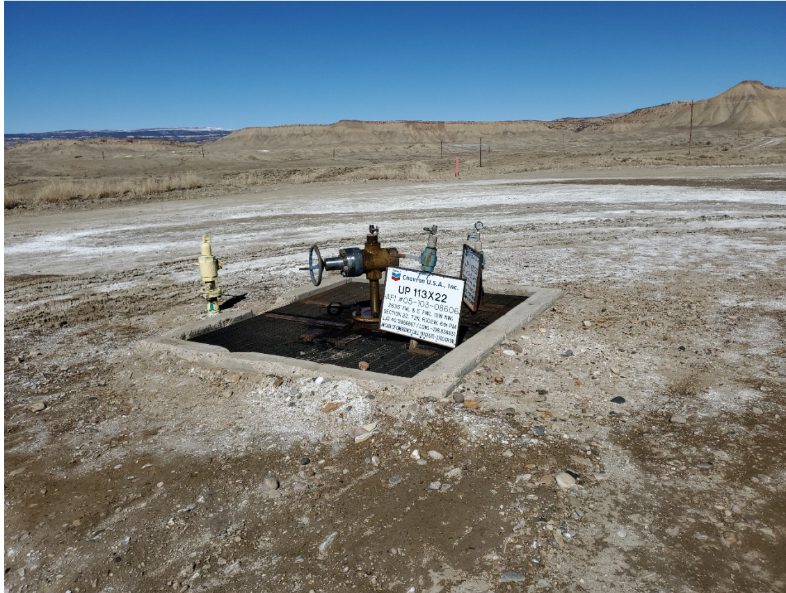
Temporarily Abandoned production wellhead. Planned UIC wellbore.
