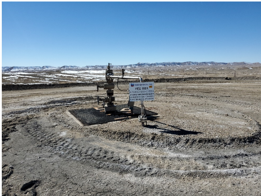
Injection wellhead
