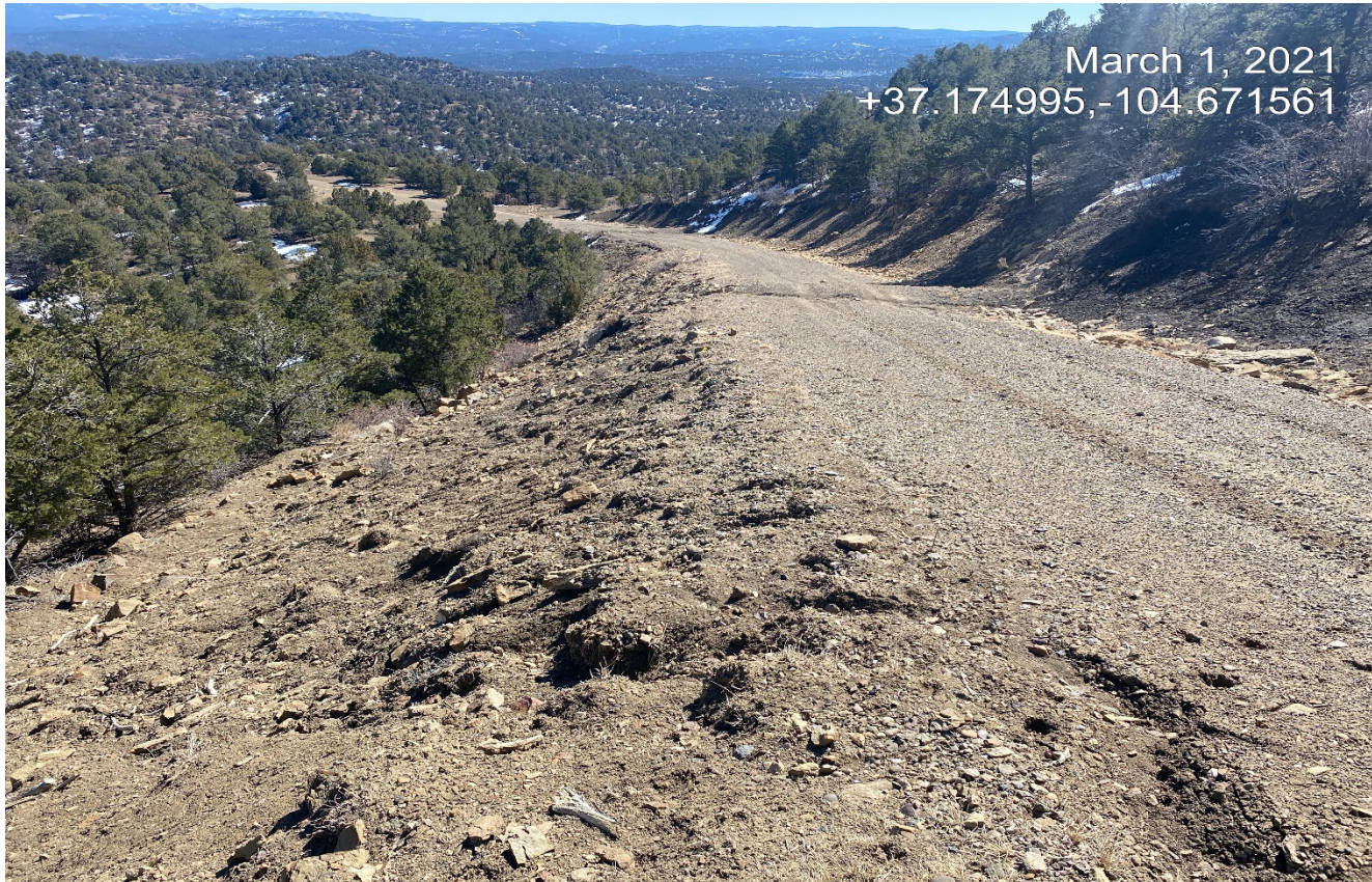
Photo 4. Facing back southeast along the access road. There is signs of erosion along the fill slope.
