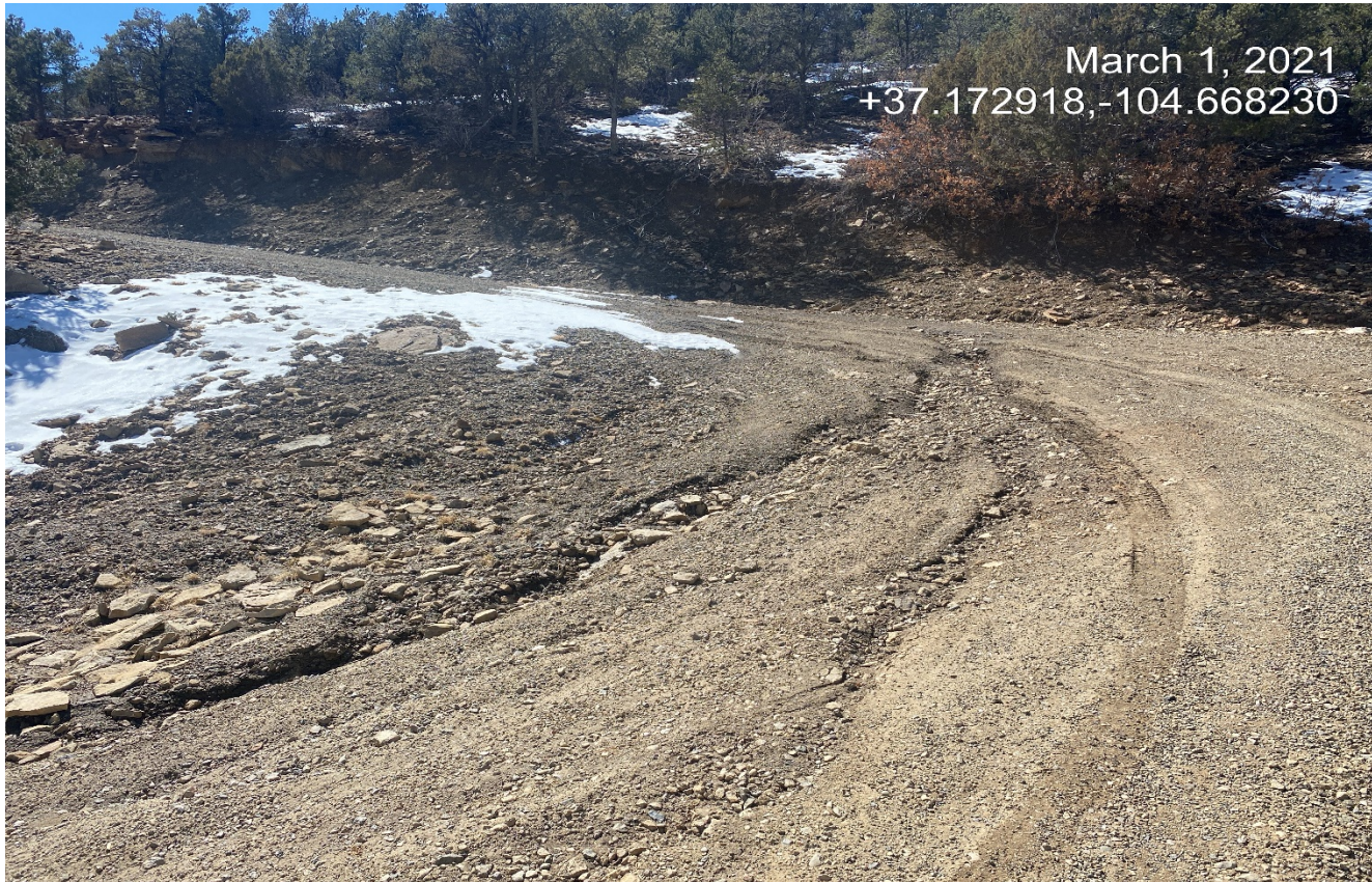
Photo 2. There is erosion along the switch back of the road. Stormwater is not being properly directed.
