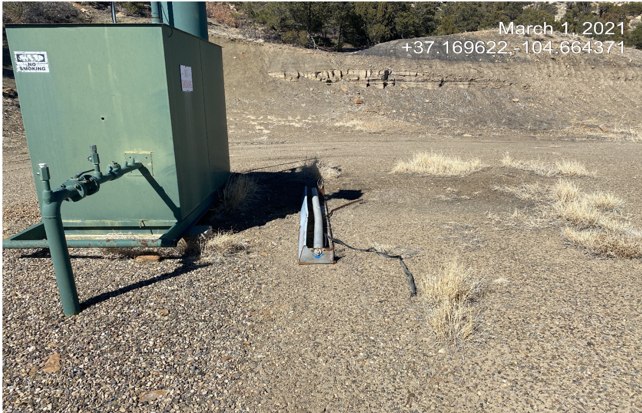
Photo 3. What appears to be a tarp roller off a dump truck lays next to the meter shed. Unused equipment needs to be removed.
