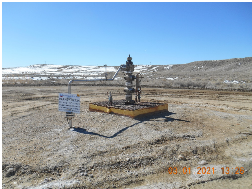
Injection wellhead
