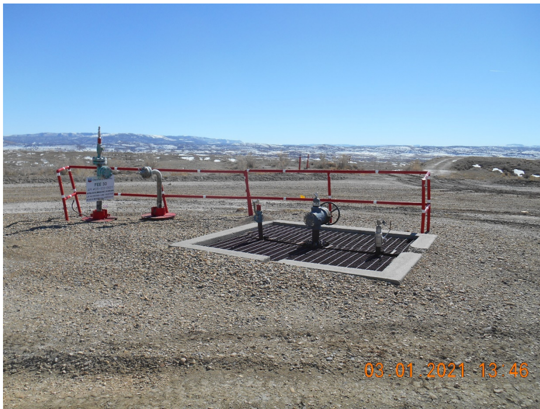
Injection wellhead – Temporarily Abandoned
