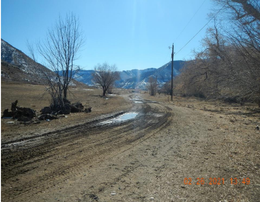
Access road shows signs of lack of stabilization BMP's in some areas (rutting is present).
