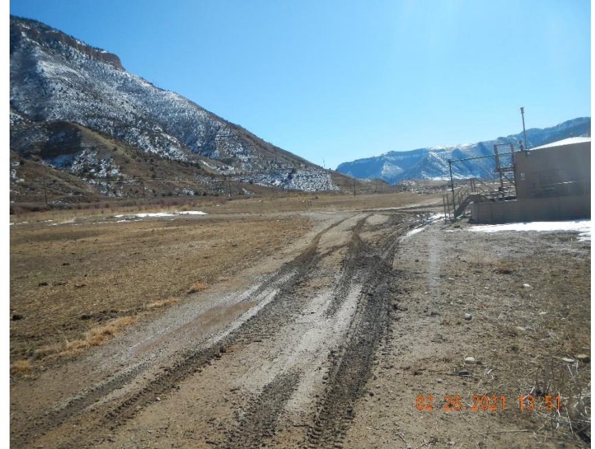
Access road shows signs of lack of stabilization BMP's in some areas (rutting is present).
