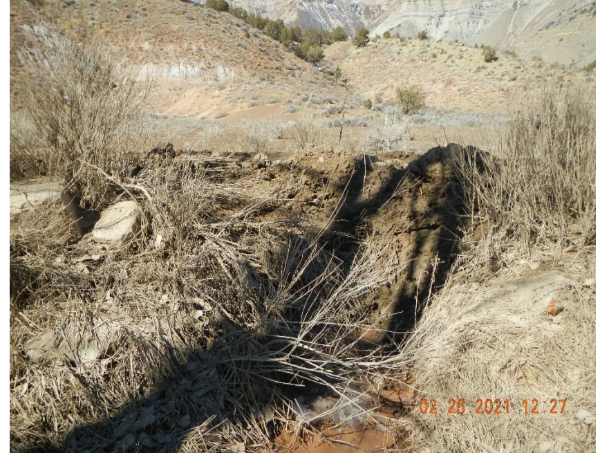
Culvert basin needs maintained.
