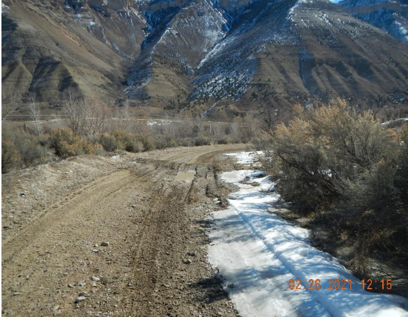
Drain crossing road. Access road shows signs of lack of stabilization BMP's in some areas (rutting is present).
