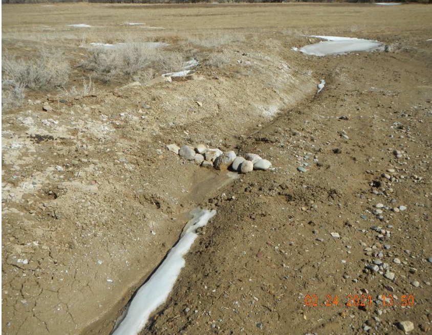
Ditch along road to lower well pad loosely compacted.
