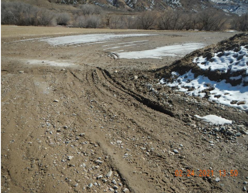
Road and location shows signs of lack of stabilization BMP's in some areas (rutting is present).
