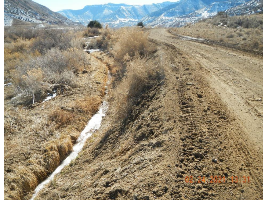
Unable to see culvert outlet. Sediment being bladed off shoulder of road.
