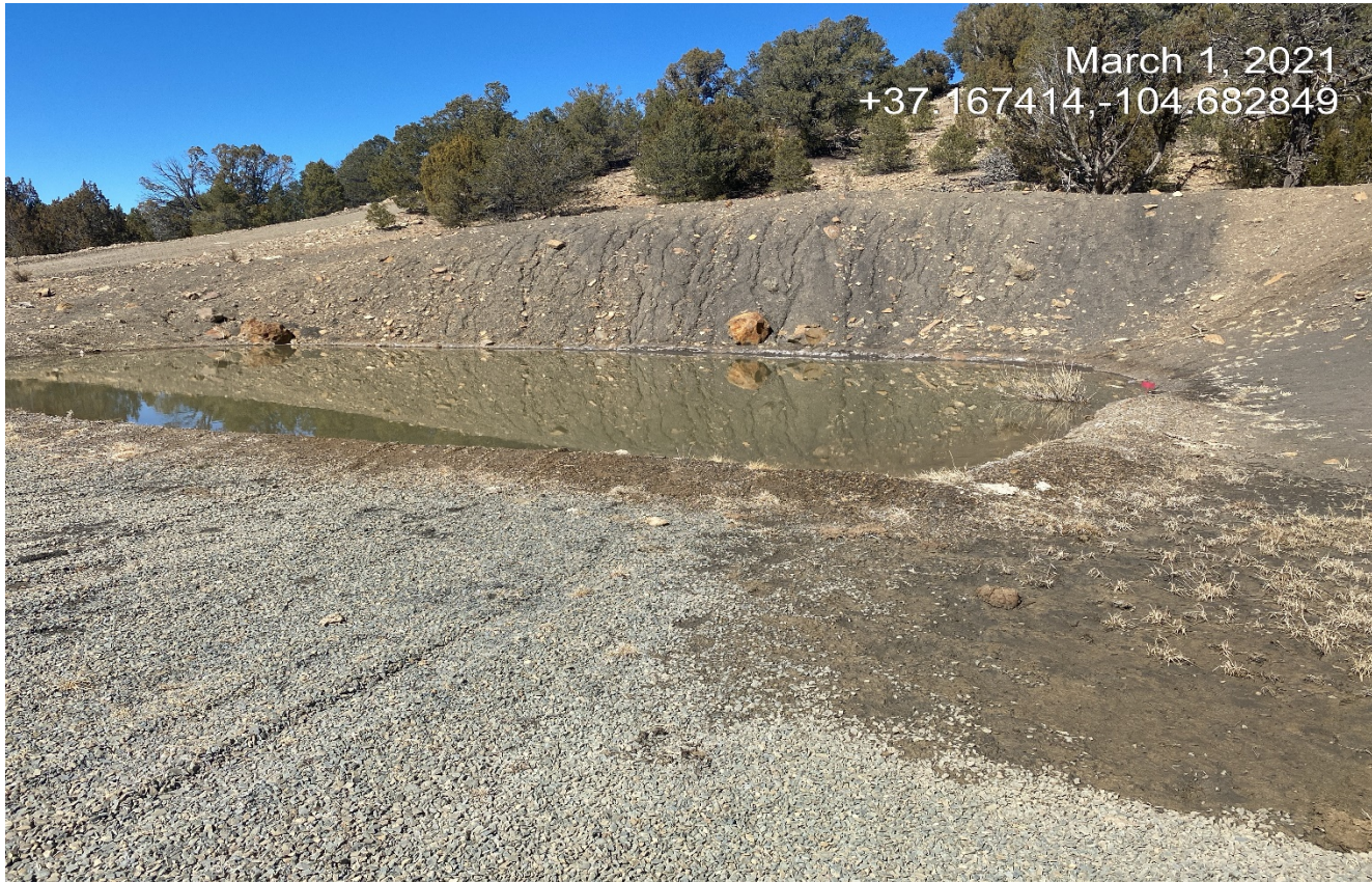
Photo 2. Water level in the pit is above freeboard and needs to be lowered.
