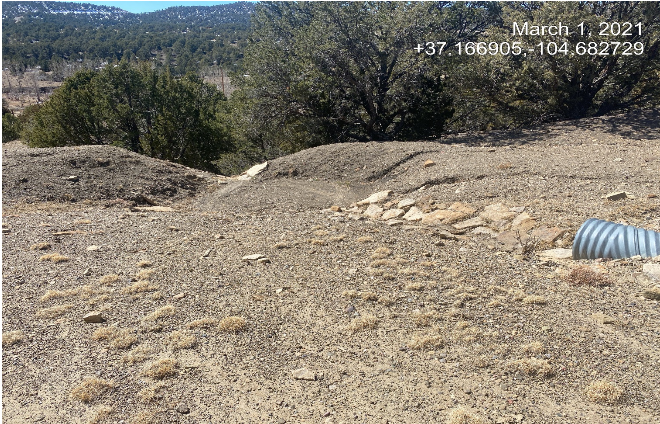
Photo 3. The sediment trap has filled in with sediment.
