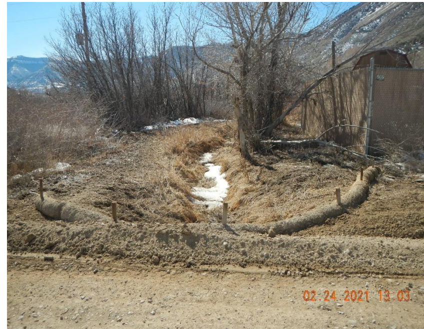
Wattle repaired or replaced.
