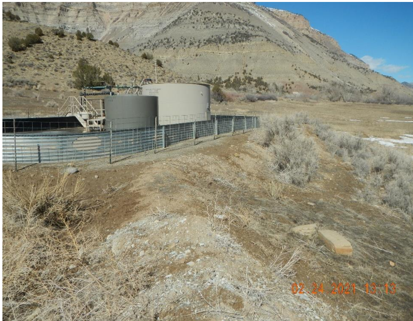
Perimeter berm behind tank battery is not consistent.
