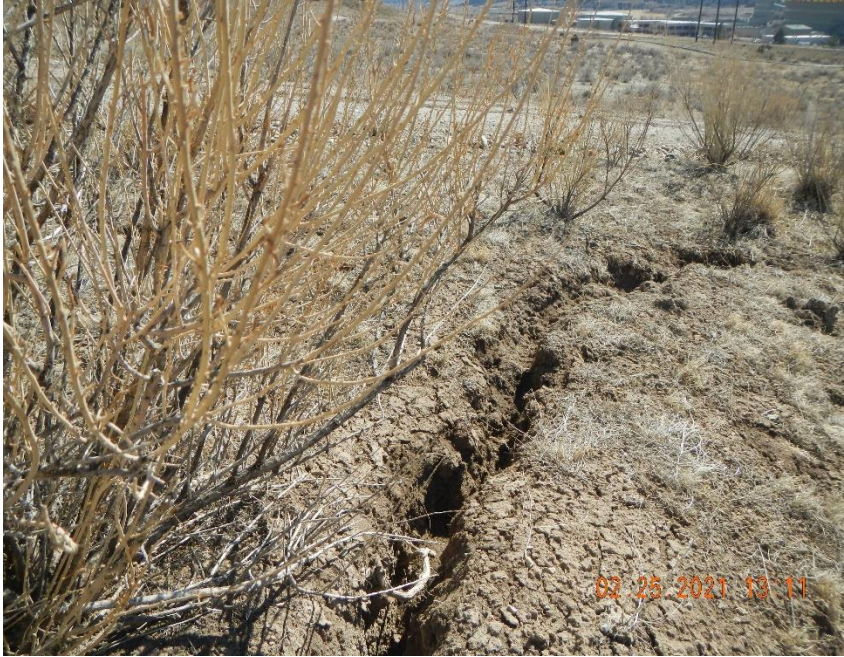
Erosion subsidence crack along up hill road into location.
