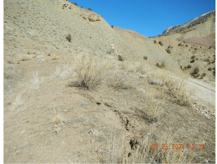
Erosion subsidence crack along up hill road into location.
