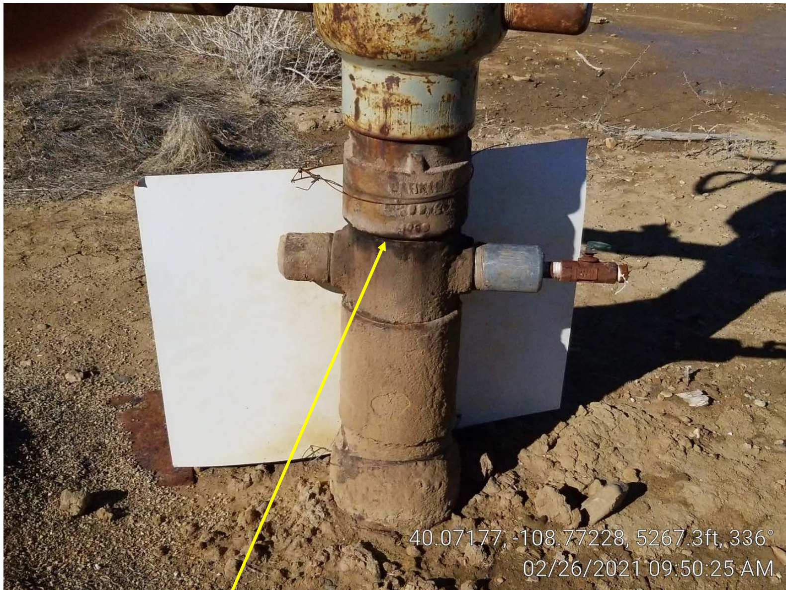
Photo 2. Well gas leak.
