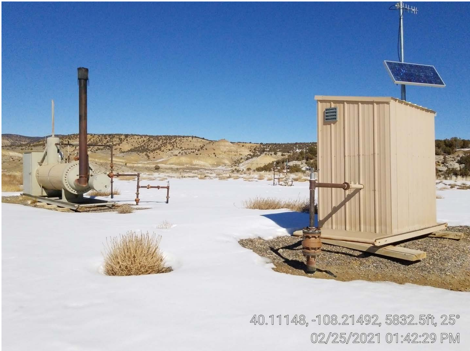
Photo 3. Separator & meter building.
