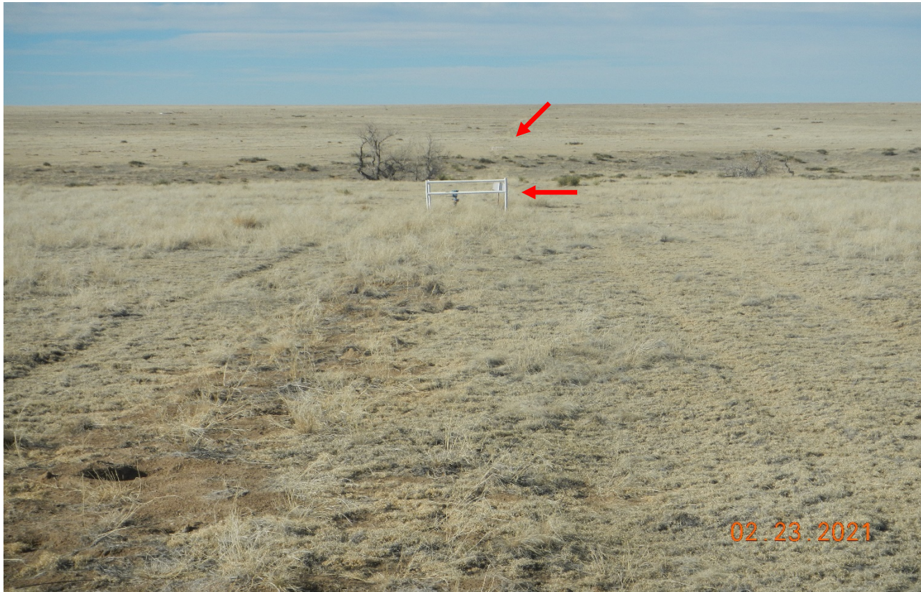
Photo 7. Facing northwest approximately 1400 ft. northwest of the location There are two pipe risers associated with the well site that have not been removed. All equipment/risers must be removed.
