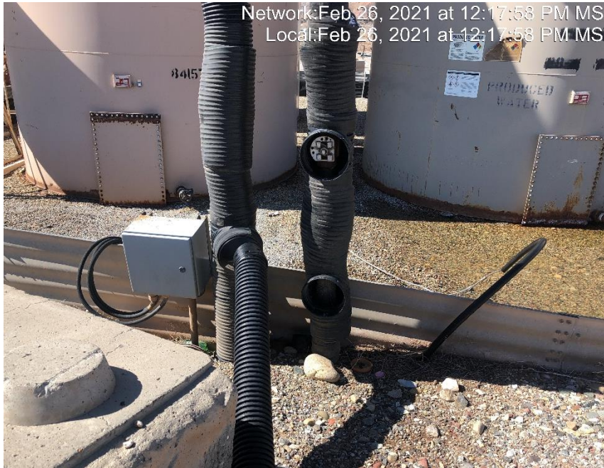
Photo #3010 Multiple places with flow line heating insulation open ended and not capped.
