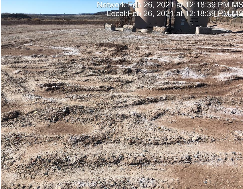
Photo #3012 Rutting present on location due to lack of stabilization.
