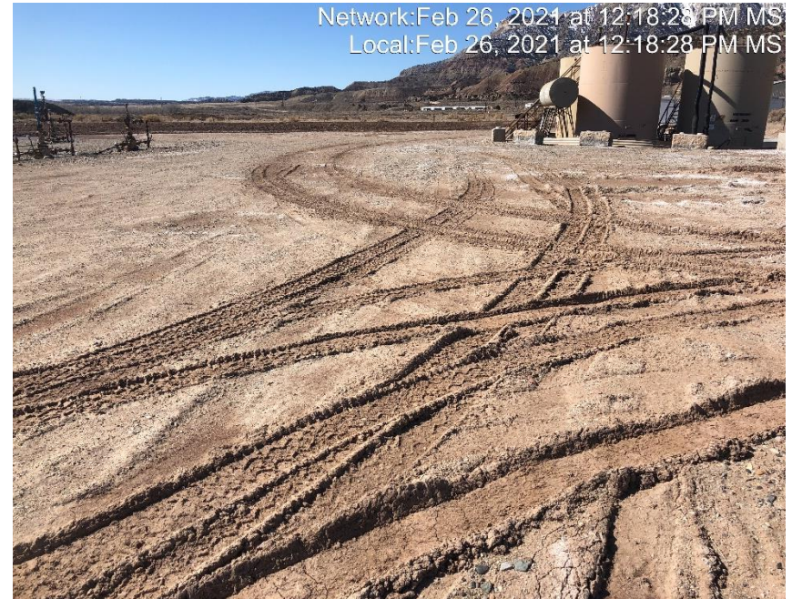
Photo #3011 Rutting present on location due to lack of stabilization.
