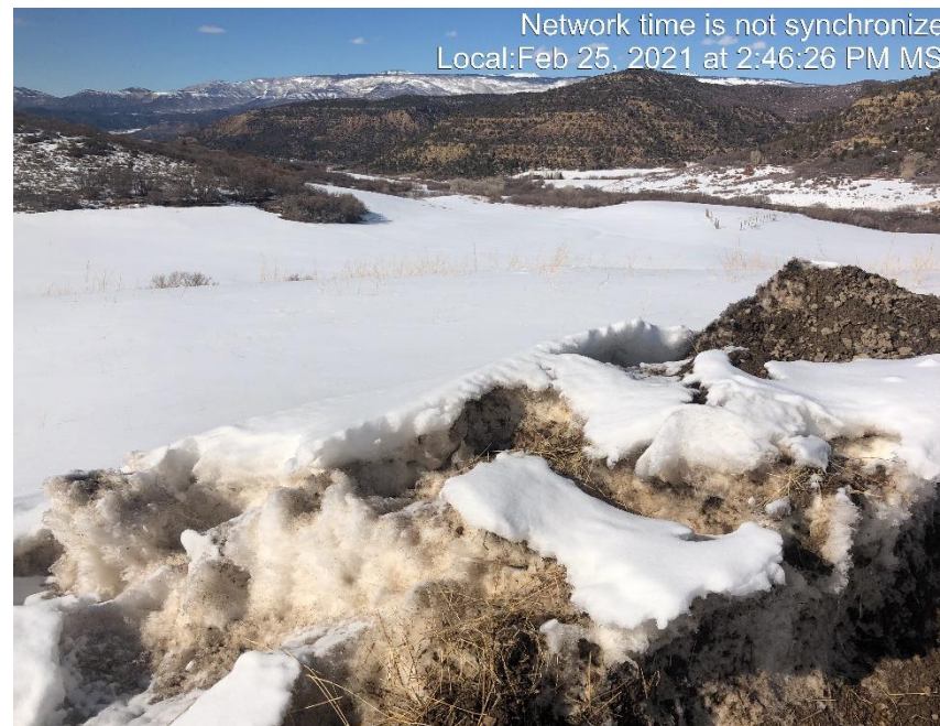
Photo #2997 No BMP's located between the edge of fill slope and Sediment pile.
