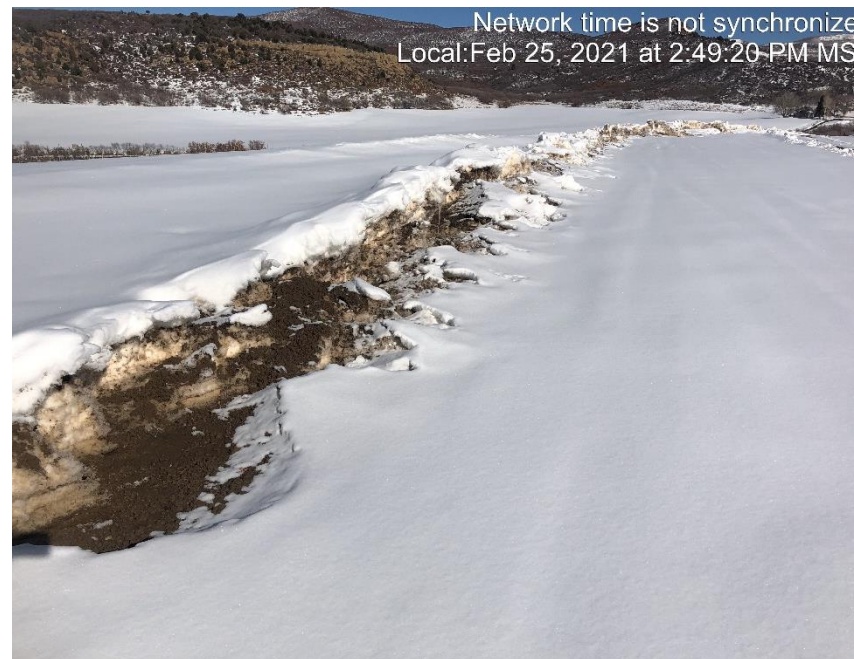
Photo #2999 Sediment has been transported off of location due to snow plowing.
