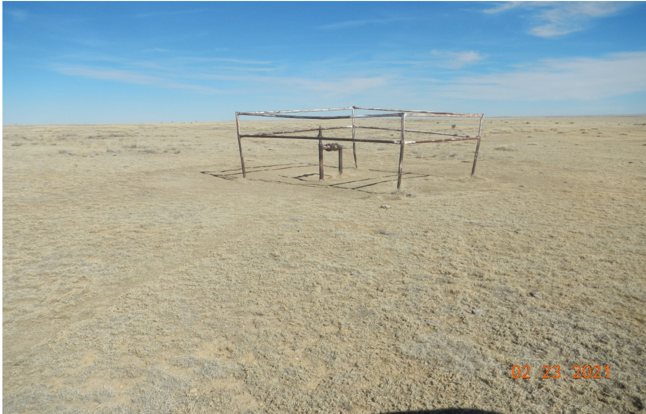
Photo 6. Another pipe riser associated with the well site was found at Lat/Long:37.87789,-102.71800. All equipment/risers need to be removed.
