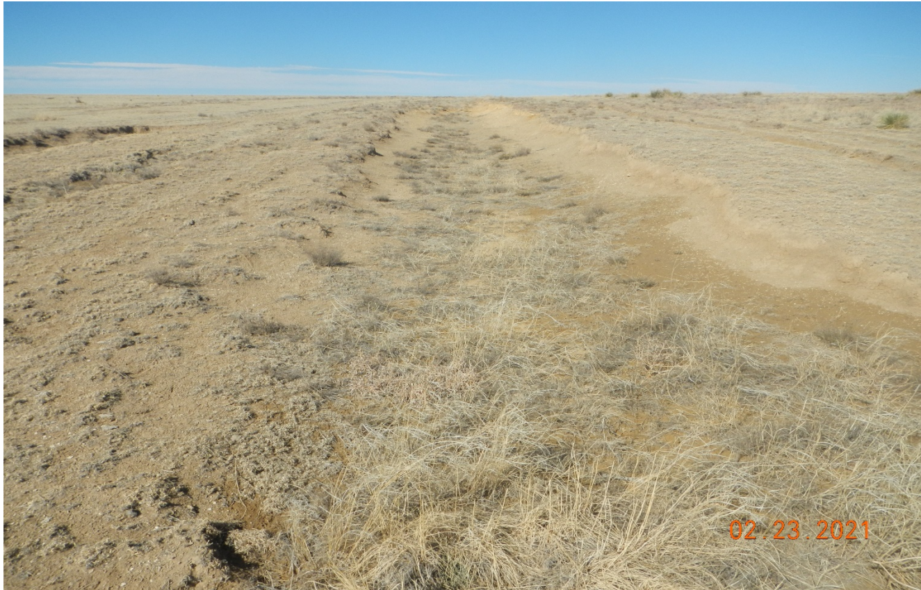
Photo 2. Facing north along the former access road at Lat/Long:37.87672,-102.72188. This area of the road has eroded and needs to be repaired and reclaimed.
