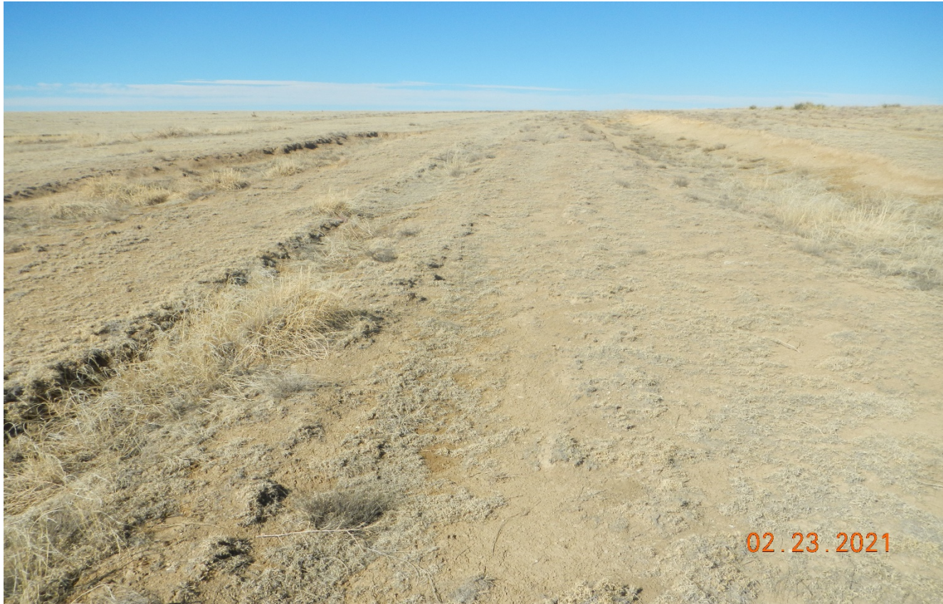
Photo 1. Facing north along the former access road at Lat/Long:37.87672,-102.72188. This area of the road has eroded and needs to be repaired and reclaimed.
