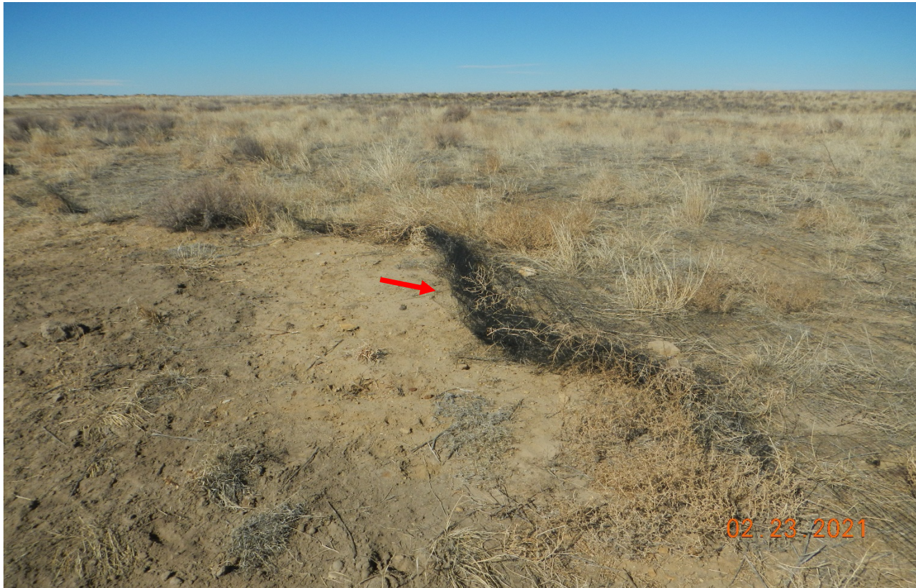
Photo 5. Facing northwest at the location where reclamation was previously performed. The plastic netting from the blanket is bunched up in areas and should be cut and removed without pulling up the vegetation.
