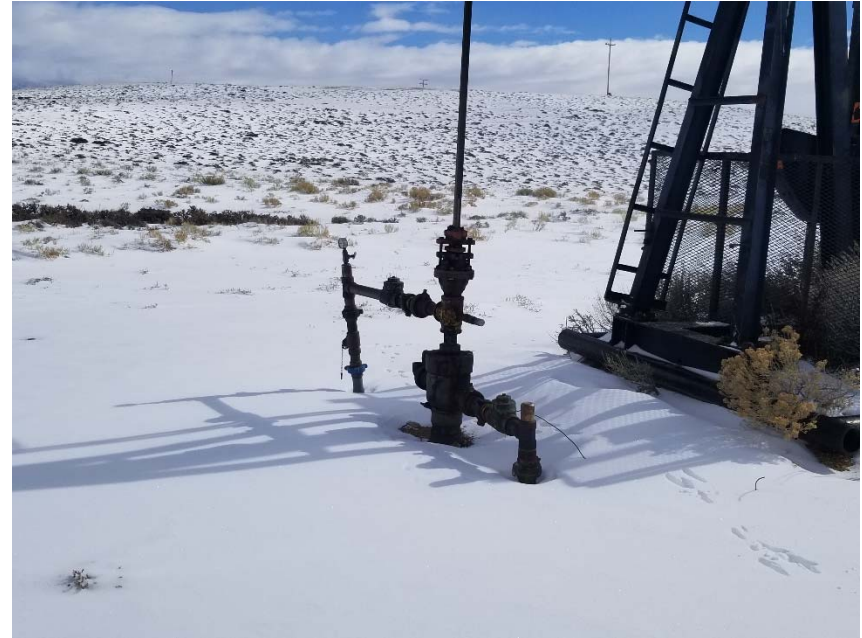
Photo 2. No bradenhead access apparent.
