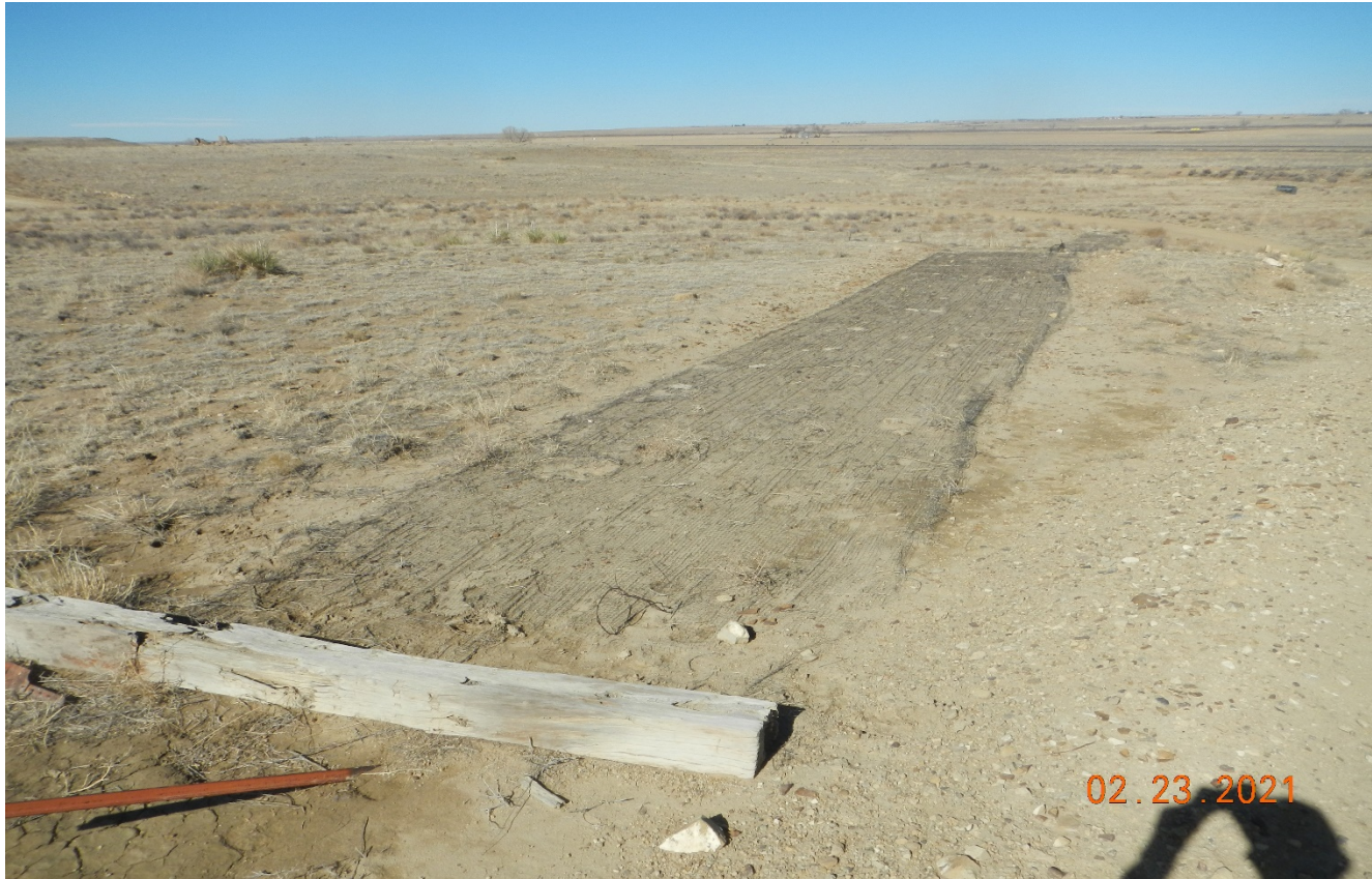
Photo 1. Facing toward the disturbance adjacent to the main road which had been previously cited. This area was repaired however vegetation has not established and the BMP's are degraded.
