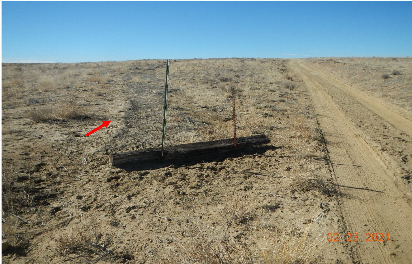
Photo 3. Facing toward the disturbance adjacent to the main road which had been previously cited. This area was repaired however vegetation has not established and the BMP's are degraded.
