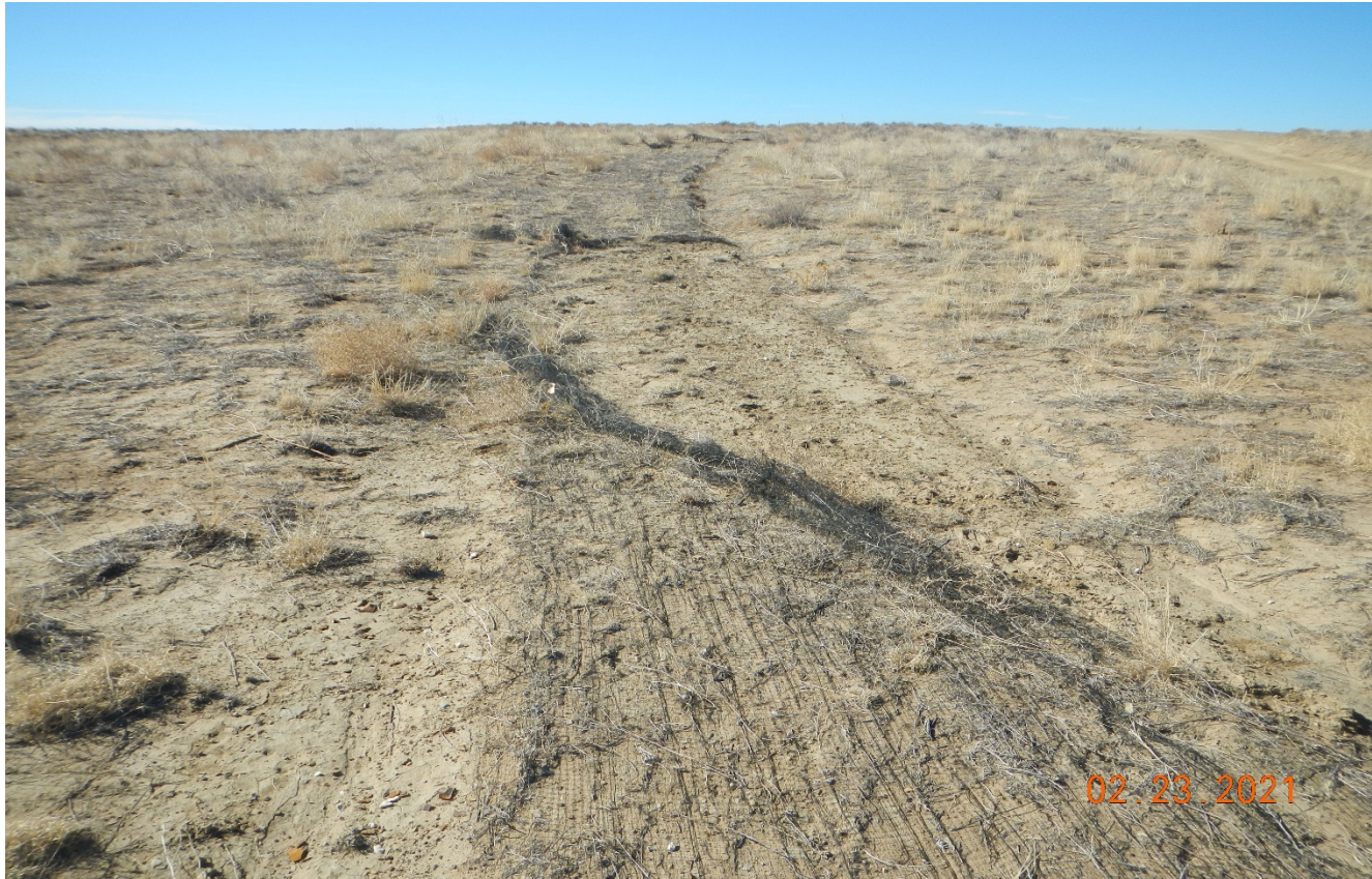
Photo 4. The netting from the straw blanket needs to be removed in areas without pulling up vegetation. Bare areas need to be reseeded.
