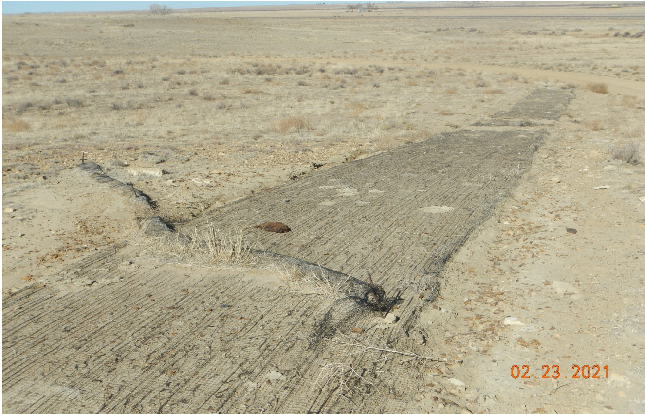
Photo 2. The wattles and straw blanket are degraded.
