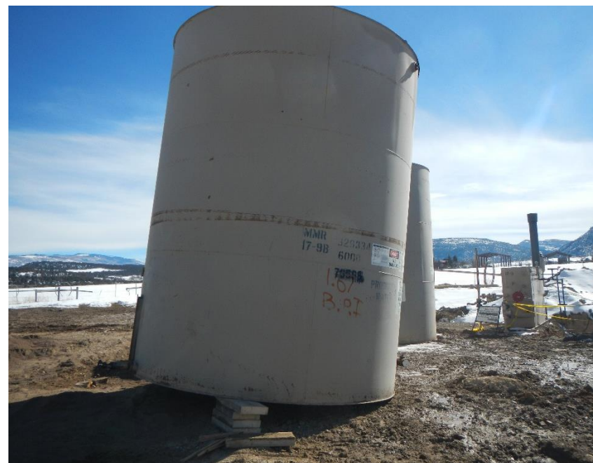
Production tanks removed from containment, and propped at an angle by wooden blocks.
