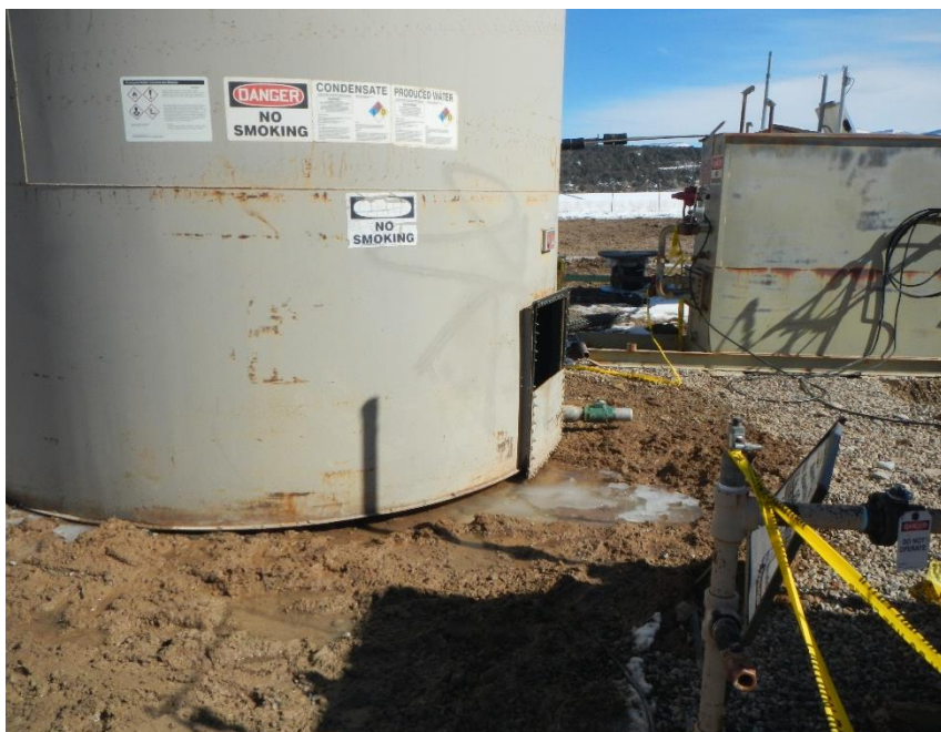
Production tank removed from containment for repairs. Manway is open, not secondary containment.
