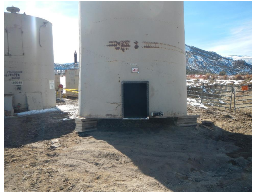
Open manway on production tanks
